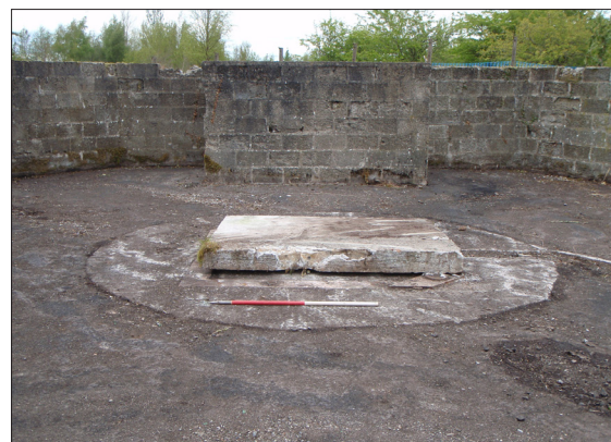
Plate 2: Battery E6, detail of emplacement after clearance.
