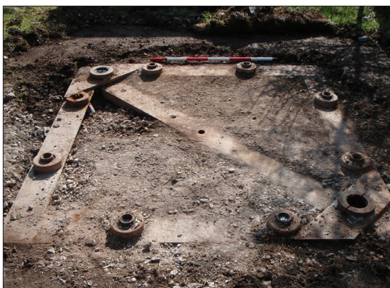
Plate 1: Battery E5, detail of footings from south.
