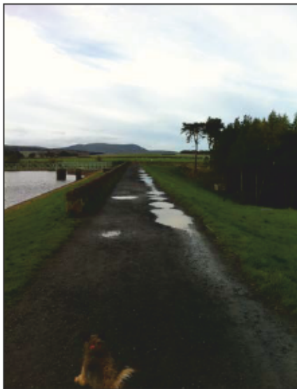
Plate 20: General view along the top of the dam, from the north-east.
