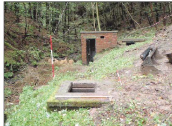
Plate 5: Building 4, brick and concrete manhole with cast-iron cover removed. Buildings 2 and 3 to rear of frame. From the SSW.
