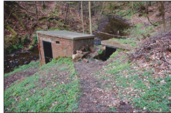
Plate 4B: Building 2 and Building 3, from the east-south-east.
