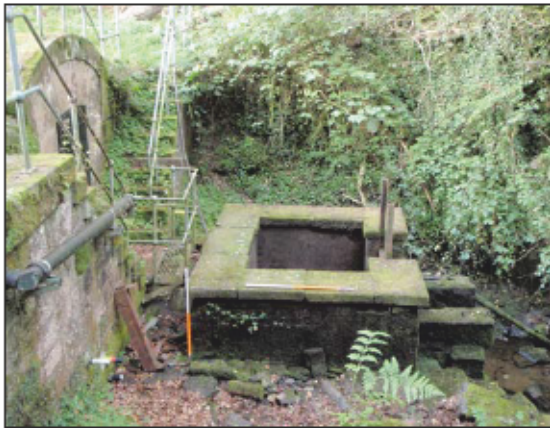
Plate 6: General view of Building 5, from the north-east.
