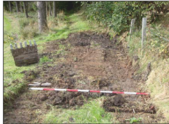
Plate 14: General view during topsoil stripping to form temporary access road.
