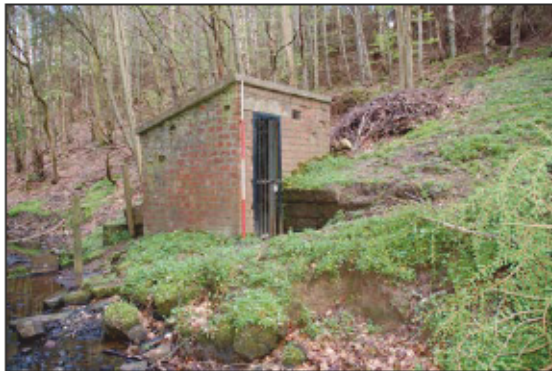
Plate 3: Building 2 with sandstone revetting wall, from the south-west.
