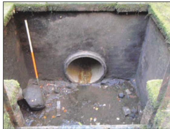
Plate 9: Inlet pipe to tank, from the north-west.
