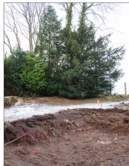
Plate 2: General shot of yew tree west of site.
