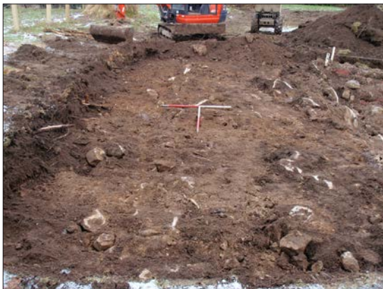
Plate 1: Shot of patio area during topsoil stripping.
