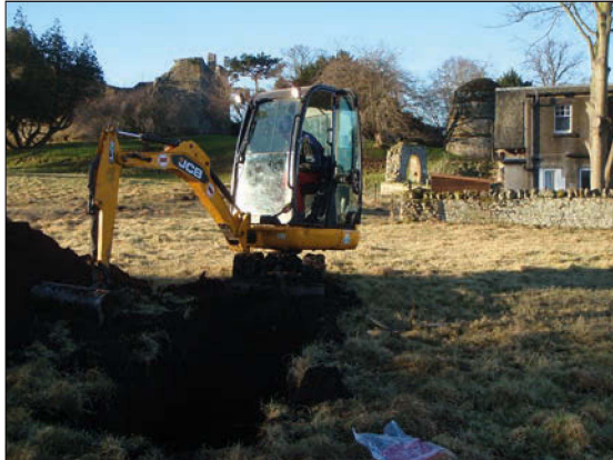
Plate 6: General view during excavation of trench 1.
