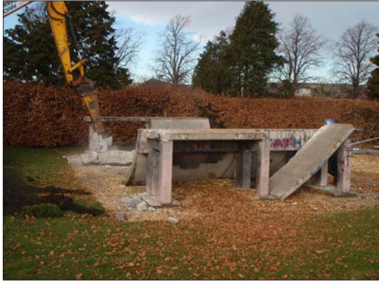
Plate 3: Skateboard half-pipe during demolition, from the south.
