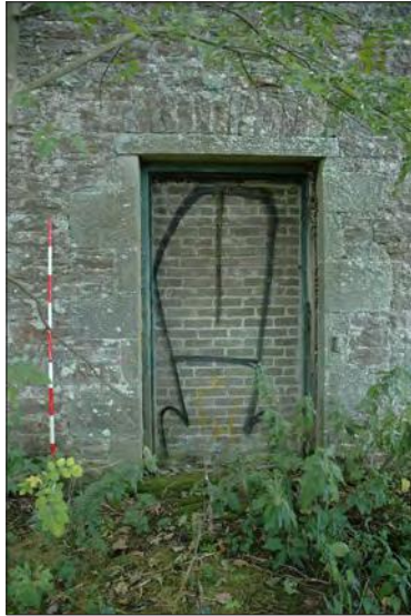
Plate 10: Doorway within south-west wall, interior elevation.
