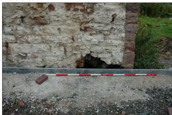
Plate 5: Detail of small blocked splayed arch.
