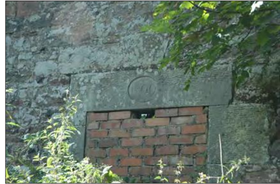
Plate 11: '1809' date inscription above south-east wall doorway: exterior elevation.
