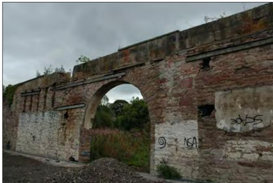
Plate 3: Entrance archway in north-west wall showing vertical vents, exterior elevation.
