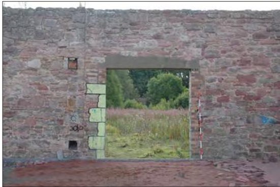
Plate 8: Entrance within west-northwest wall.
