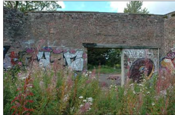
Plate 9: West-southwest wall internal elevation.
