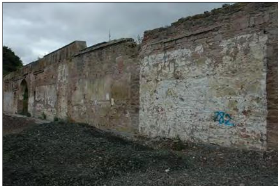
Plate 6: Locations of later 'lean-to' structures, north-west exterior elevation.
