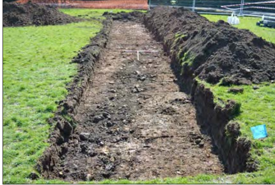
Plate 3: Rubble drain Trench 5.
