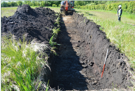
Plate 3: Detail shot of trench 13 showing deep intermediate layer.
