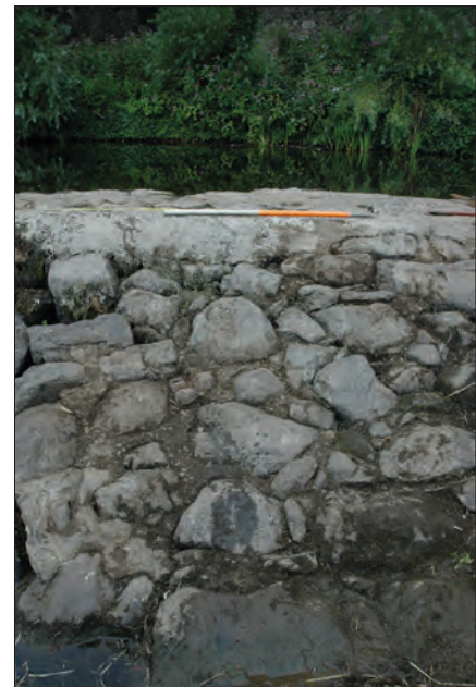
Plate 2: View of the fabric of the spillway after vegetation strip showing roughcast concrete pointing 004, from the SE.
