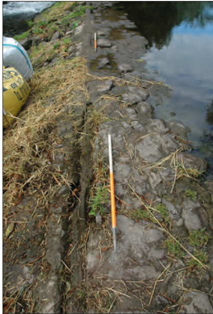
Plate 3: Degraded timber beam 002 left of near ranging rod with later replacement concrete blocks 003 left of far ranging rod, from the NE.
