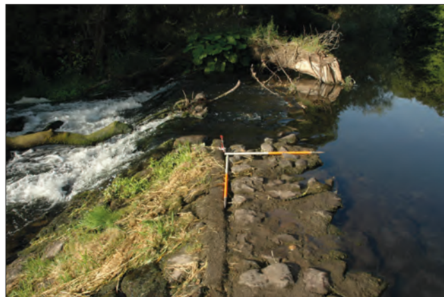
Plate 5: Breached section of the weir with thick roughcast concrete screed 004 consolidating the top of weir, from the NE.
