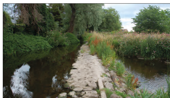
Plate 9: south-east section of the weir after consolidation work.
