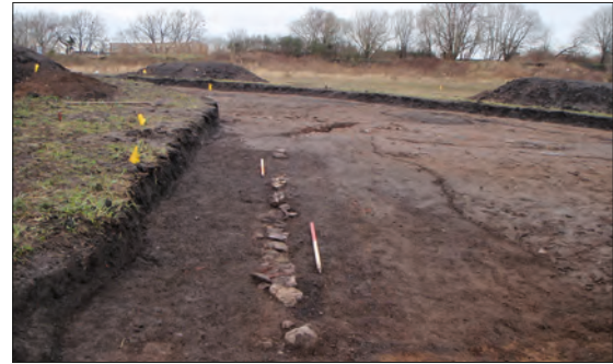
Plate 61: Kerb 2014 at the north end of track 2054, to the immediate south of the area of hard standing in the north-west corner of Phase 2.
