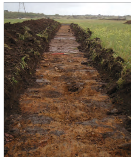
Plate 41: Deposits 4900 and 4901 in trench 49, from the SW.
