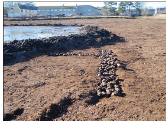
Plate 59: Rubble drain/soakaway 1025, from the north-east.
