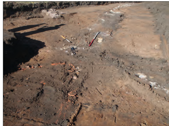
Plate 2: Culvert 1201 after expanding trench 12, tile drains visible entering the SW extent of culvert with tile drain 1209 and stone setting 1200 aligned diagonally from top left to bottom right of frame.
