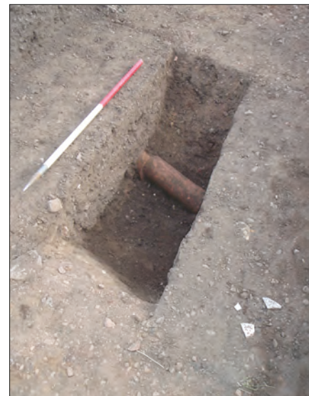
Plate 8: Ditch cut and fill 2001/2200 containing a horseshoe shaped tile drain at the base of the cut. This was a continuation to the east of the ditch that contained culvert 2403 in trench 24, view from the north.
