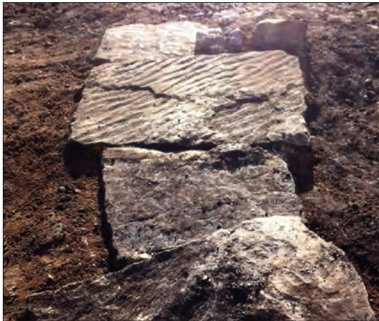
Plate 65: Culvert 2051, from the north-east.
