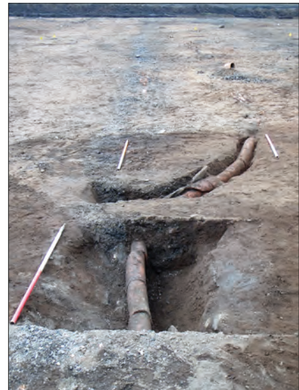
Plate 64: Drain 2082, from the north-west.
