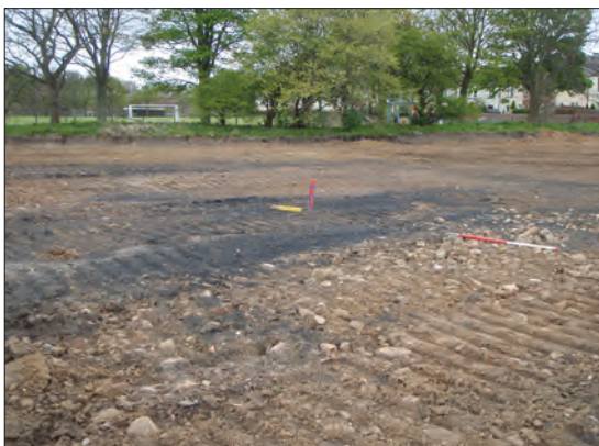
Plate 67: Mineshaft [5000] beyond the red peg with sandstone rubble deposit [5002] below ranging rod and coal dross deposit [5001] spread around mineshaft, from the east.
