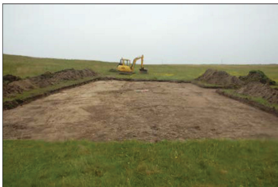
Plate 1: Plot 1 stripped, from the south-east.
