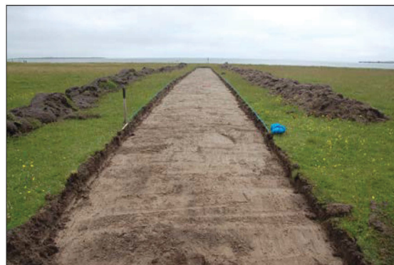
Plate 2: Access road stripped, from the north-west.
