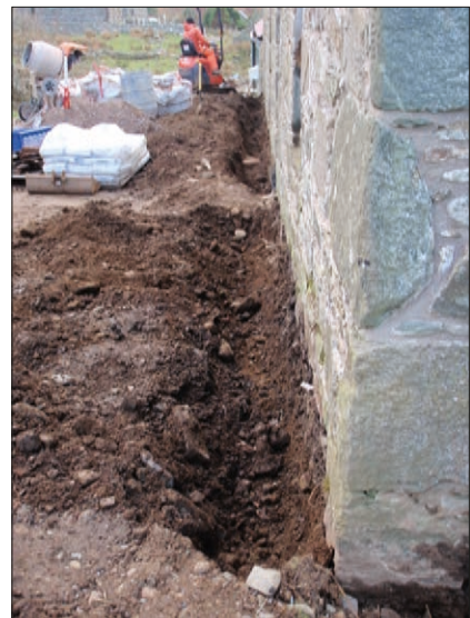
Plate 3. Trench along the east facing wall of barn B.
