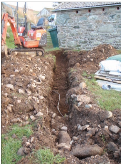
Plate 2. North west soakaway, post excavation.
