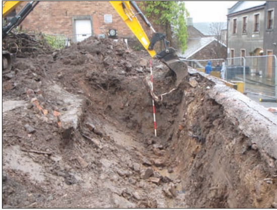
Plate 3: Removal of overburden.
