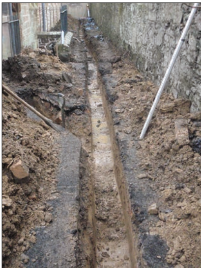
Plate 1: Northern drainage trench, from the east.
