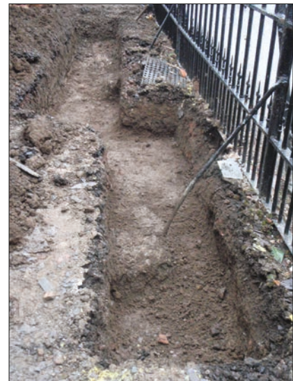
Plate 2: Southern foundations, from the west.
