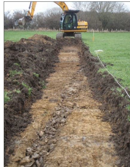
Plate 2: Stone filled rubble drain.
