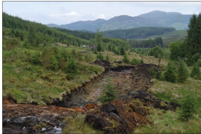
Plate 1: General view of the pipeline easement, looking towards the homestead, at the south-western end of the monitored area. Areas of deep peat can be seen in the south-east facing (uphill) section of the trench.
