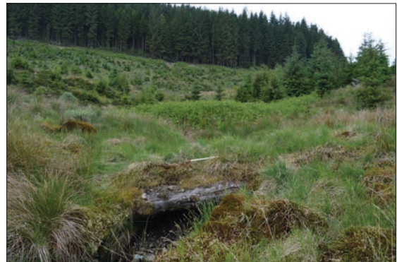
Plate 17: Tree trunks forming a bridge to carry the track over the unnamed burn at Big Bruach Caoruinn homestead.
