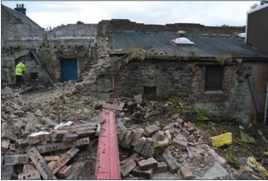
Plate 10: East facing elevation of the earlier mill building with blocked opening and later brick work and a fragment of the later sandstone built extension abutting the south side of the gable wall.
