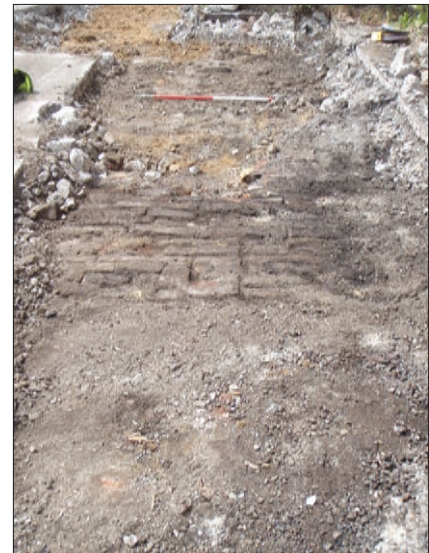
Plate 28: Partially cleaned brick and cobbled surface 201 centre of frame with possible track remnant or hard standing 200 below ranging rod, in trench 2, from the east.
