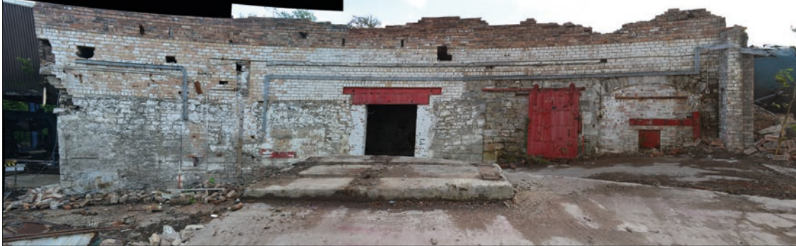
Plate 6: Composite photograph of west facing external elevation of earlier sandstone mill building below 20 th century brick, the later sandstone built extension abuts the south end of the mill building wall beyond the right hand side of the open doorway. (Image slightly distorted by image manipulating software)
