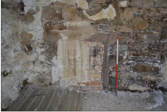
Plate 16: Blocked fireplace in north facing elevation gable wall.
