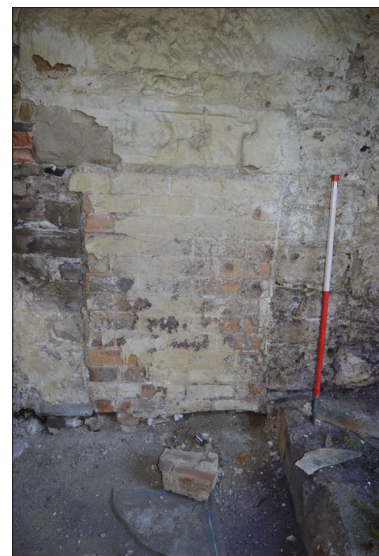
Plate 15: Blocked fireplace in north facing elevation gable wall.
