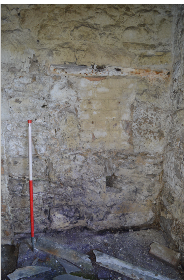
Plate 14: Blocked wall press in north facing elevation gable wall, wooden lintel visible above whitewashed brick blocking.
