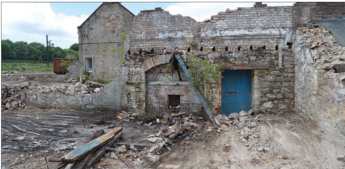
Plate 9: East facing internal elevation of later sandstone extension abutting gable end of earlier mill building right of frame.
