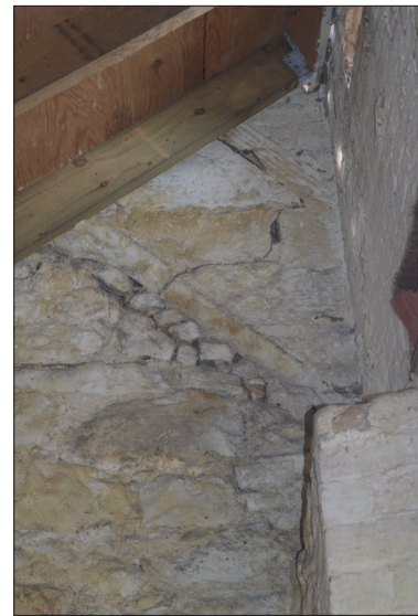
Plate 13: Detail of the roof scars associated with different phases of construction.
