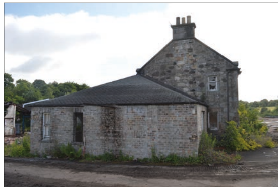
Plate 5: West facing elevation of the mill house with later brick extension.
