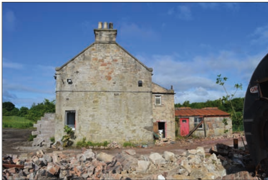
Plate 3: East facing elevation of mill house with later brick extensions abutting the north, rear elevation of the property.
