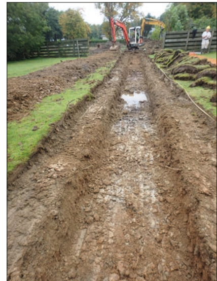
Plate 3: Subsoil north end of service trench.
