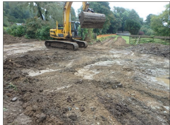
Plate 5: Eastern end of site post-topsoil removal.
