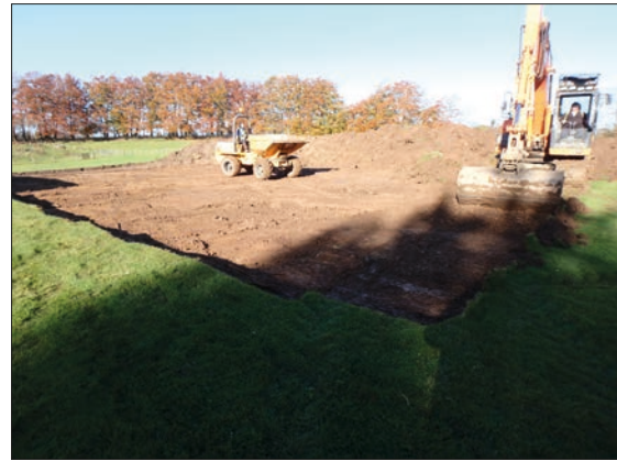
Plate 4: Post-excavation south end of site.
