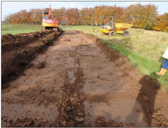
Plate 3: Post-excavation north end of site.
