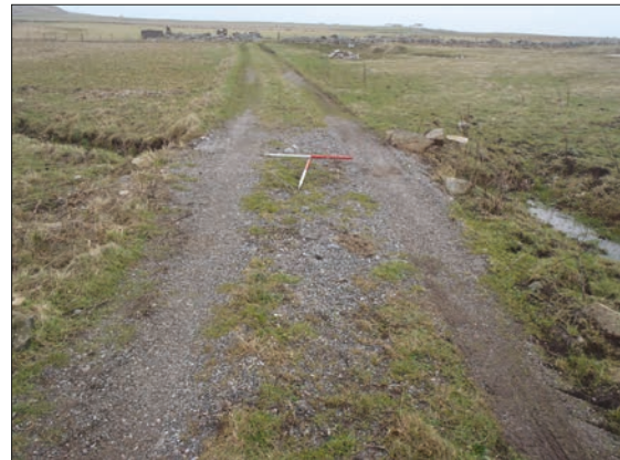
Plate 3: Existing built up access road with stone chips/gravel.
