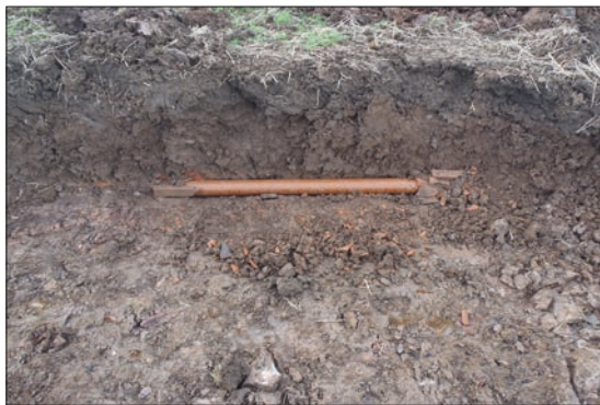
Plate 3: Repaired field drain trench 1.
