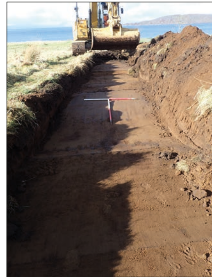
Plate 2: Working shot during topsoil strip of the new bund site.
