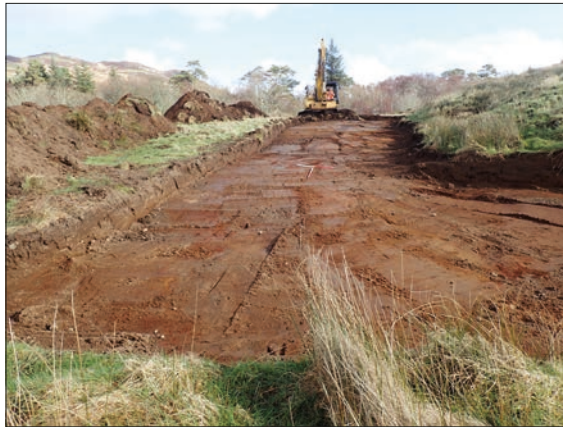
Plate 1: SW area of the site post-excitation.
