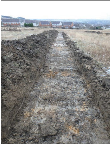
Plate 1: Trench 45, from the north east.
