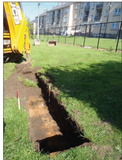
Plate 2: Test pit 101, from the west.
