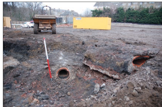
Plate 2: Redundant sewer pipe
