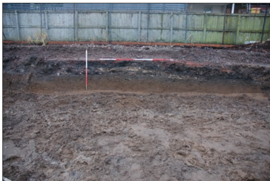
Plate 1: Overburden and soil deposits at open area excavation
