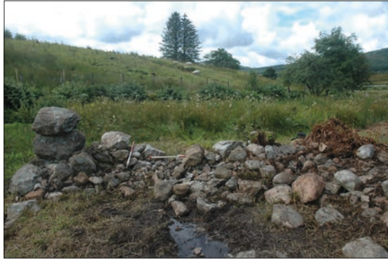
Plate 23: Collapsed stone at western wall, building U
