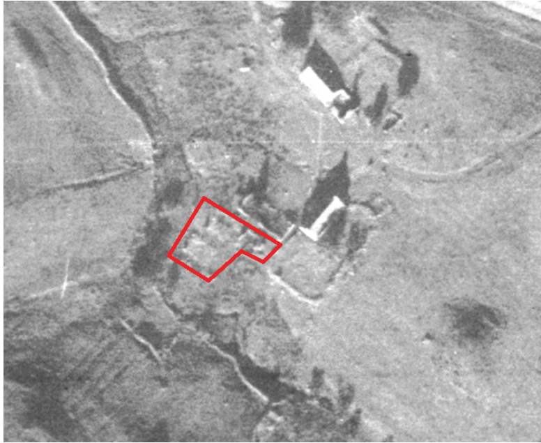
Plate 3: 1946 RAF aerial photograph with buildings T and U highlighted.
