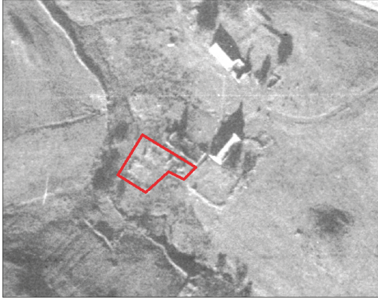
Plate 3: 1946 RAF aerial photograph with buildings T and U highlighted
