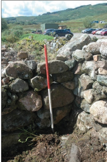
Plate 16: West partition wall 013, building T
