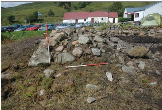
Plate 14: Corner and foundation stones in southern wall, building T
