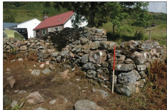
Plate 15: Foundation stone in south wall, building T
