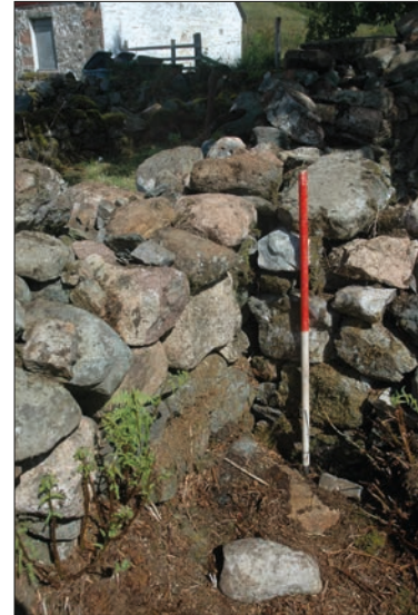
Plate 17: East partition wall 014, building T
