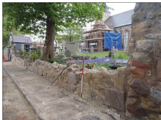
Plate 1: View of the wall after removal of upper courses, prior to archaeological monitoring commencing, taken from the east
