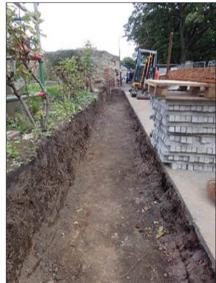
Plate 3: View of fully excavated foundation trench from the west
