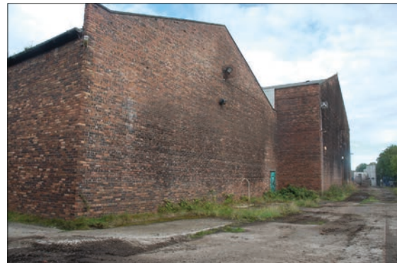
Plate 2: Original brick constructed warehouses from the south.
