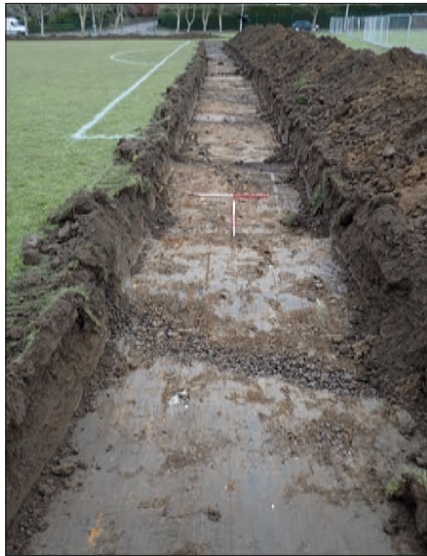
Plate 1: Trench 7. View from the south
