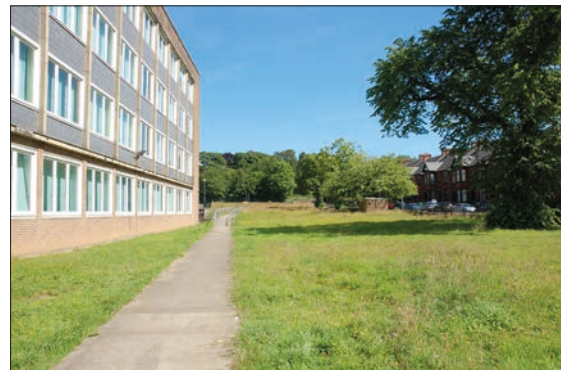
Plate 3: Grassed area at the east of the Site.
