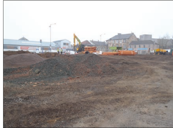
Plate 1: General view of site
