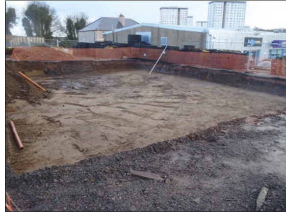
Plate 3: Natural deposit 004 in area 4 (attenuation tank location)
