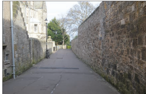
Plate 2: Butts Wynd viewed from south.
