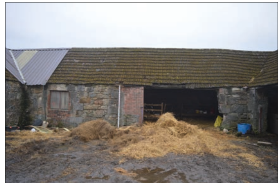
Plate 4: Repair to south exterior wall of North Range
