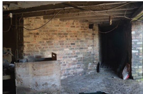
Plate 19: Brick wall in large room of farmhouse
