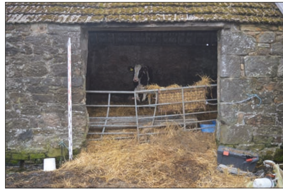
Plate 10: East wall of West Range showing wooden lintel over doorway
