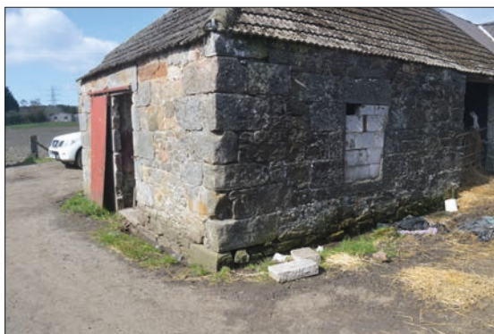
Plate 8: East wall of West Range showing blocked window and doorway
