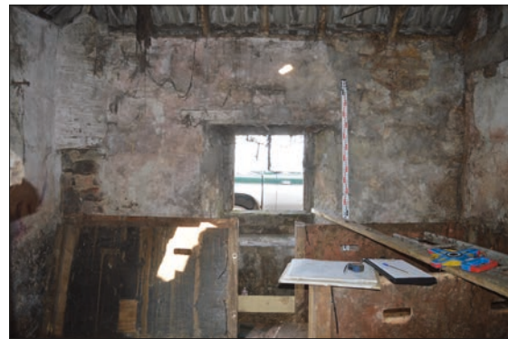
Plate 7: Internal window on west wall of West Range, room 1
