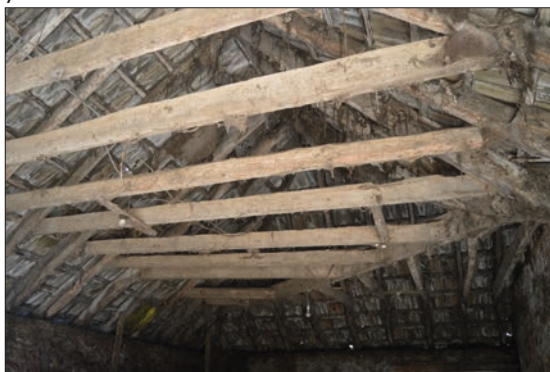
Plate 16: A-frame roof
