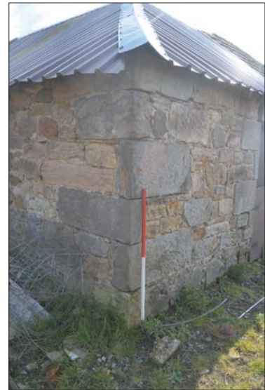
Plate 2: Quoin stones at north-west corner of steading
