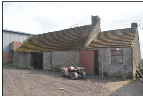
Plate 17: North exterior wall of farmhouse
