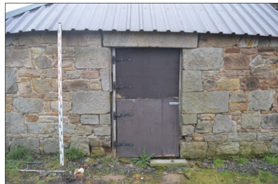
Plate 12: West wall of West Range showing door
