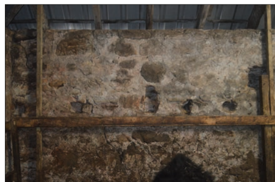
Plate 13: Beam slots at southern end of North Range
