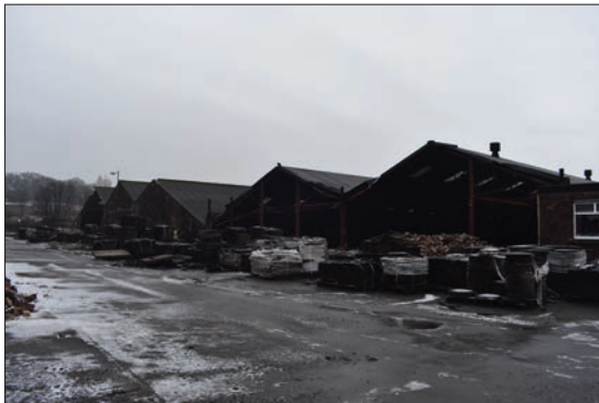
Plate 3: General view of the surviving warehouse (CHS 4) from west.
