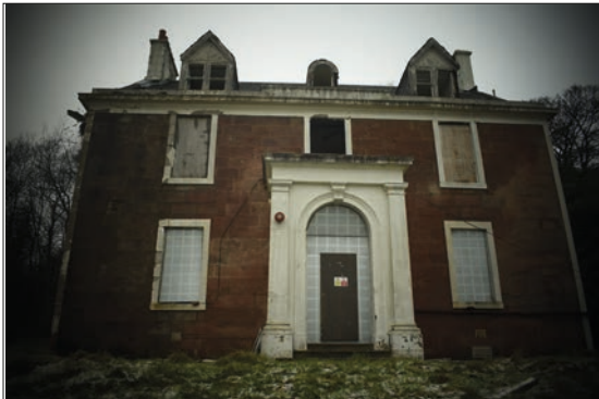
Plate 1: General view of front façade of Carsebridge House (CHS 1) from north.
