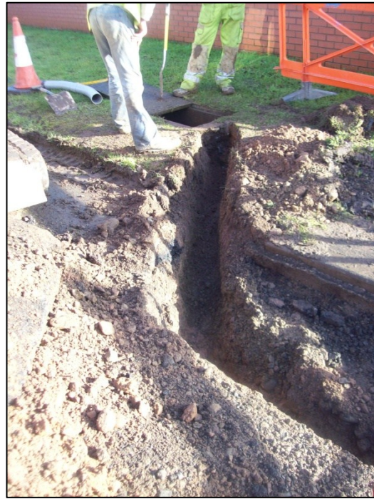
Figure 3. Machine cut trench through tarmac Figure 4. Connection to a BT junction box
