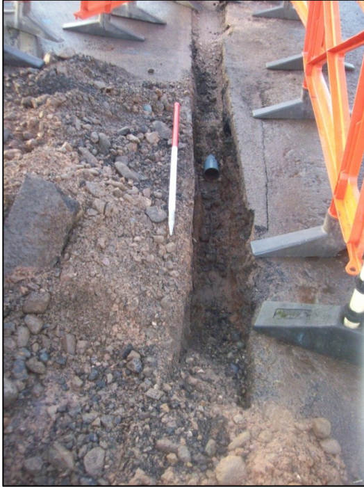
Figure 3. Machine cut trench through tarmac Figure 4. Connection to a BT junction box
