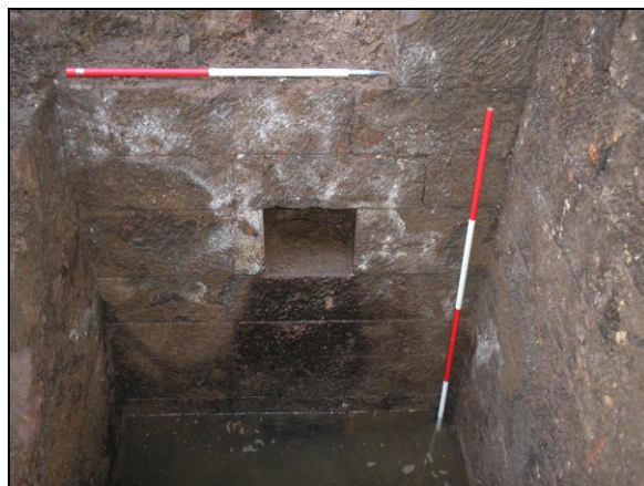
Figure 10. North wall of wheel-pit
