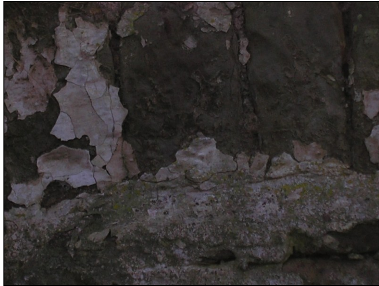
Figure 17. Stone voussoir in Building 4
