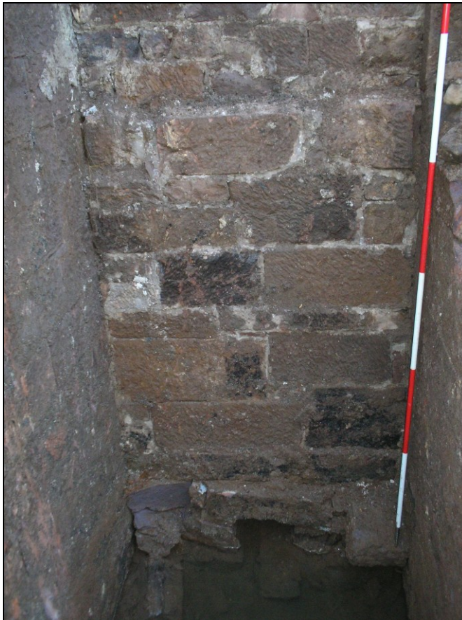
Figure 13. South elevation 2 of wheel-pit
