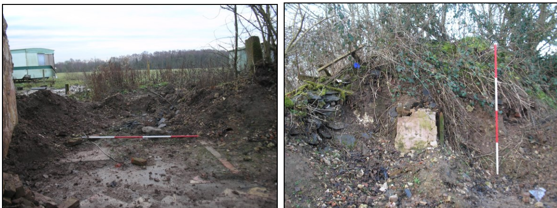
Figure 9 and 10. Reduced southern clay dabbin wall and western clay dabbin wall
