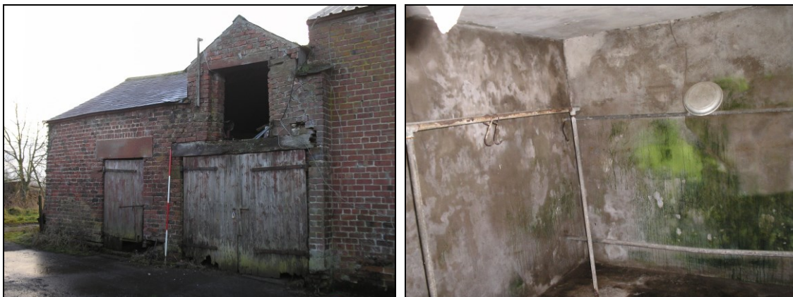
Figures 18 and 19. Eastern brick offshoot and interior showing a cattle shed
