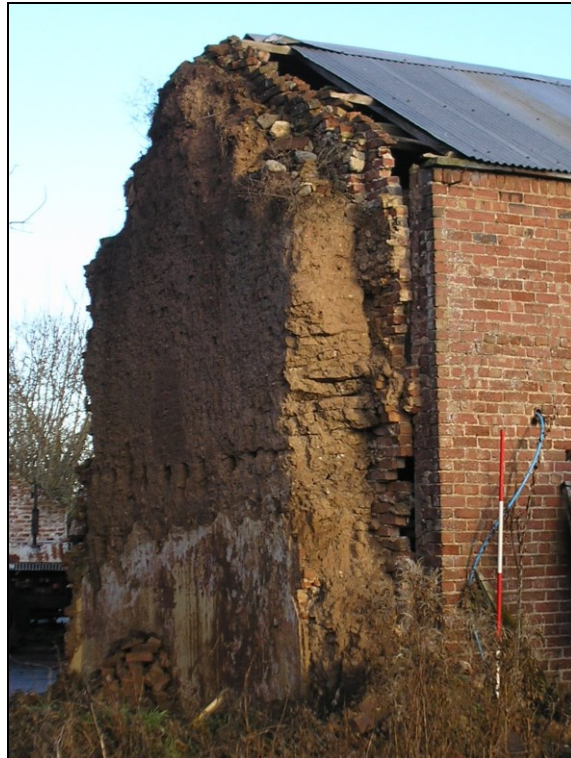
Figure 21. Eastern gable with applied brick skin
