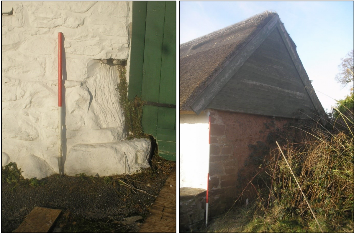
Figure 9. Cruck blade emerging through the wall Figure 10. Clay wall, eastern elevation
