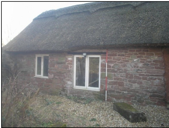
Figure 14. Rear elevation of the cottage
