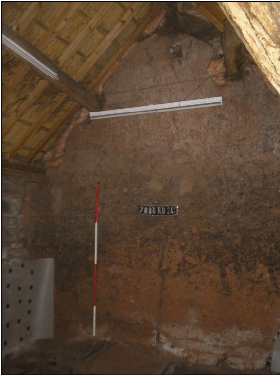
Figure 19. Clay wall eastern gable end.
