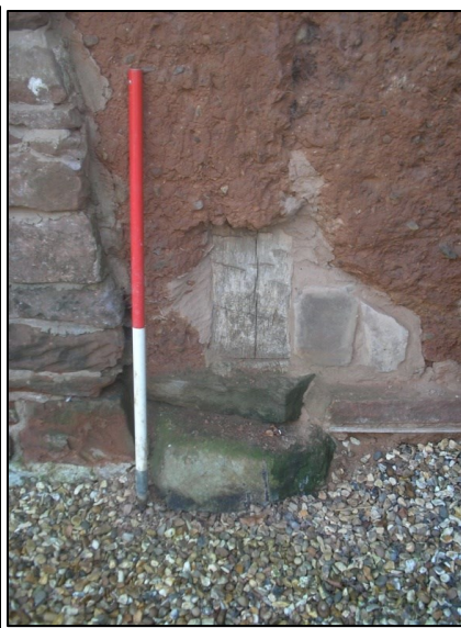
Figure 13. Base of cruck blade detail
