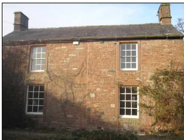
Figure 28. Bluebell House, south elevation
