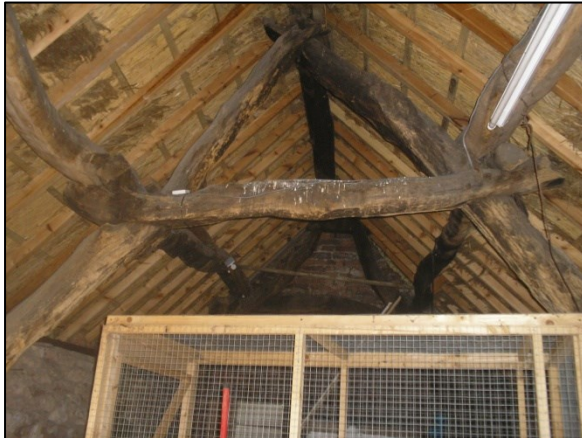
Figure 24. Eastern roof truss within cottage
