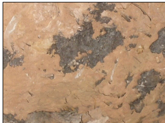
Figure 22. Detail of clay wall fabric
