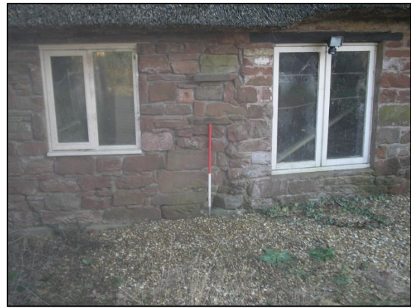
Figure 15. Interface, phase 2 and 3 stonework
