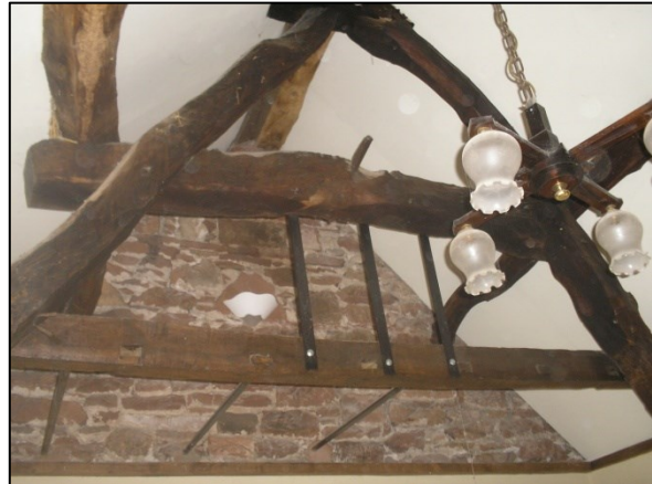
Figure 25. Western roof truss within snug
