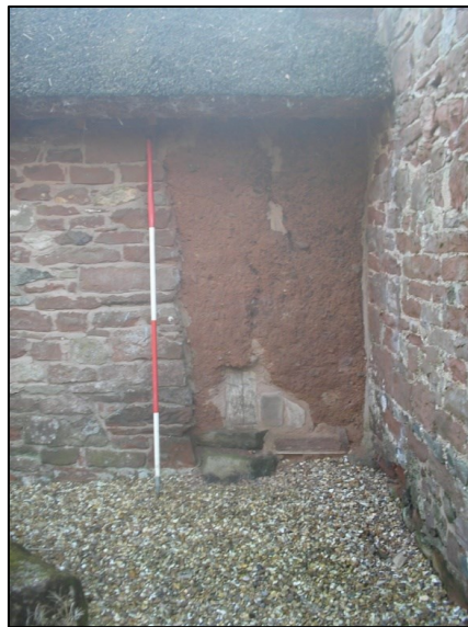
Figure 12. First phase clay wall
