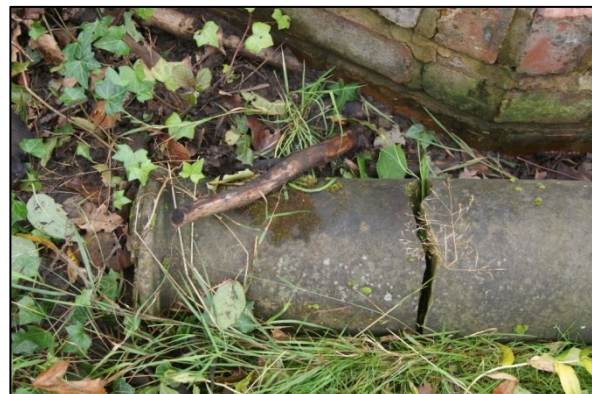
Figure 16. Broken head of the pillar with beading
