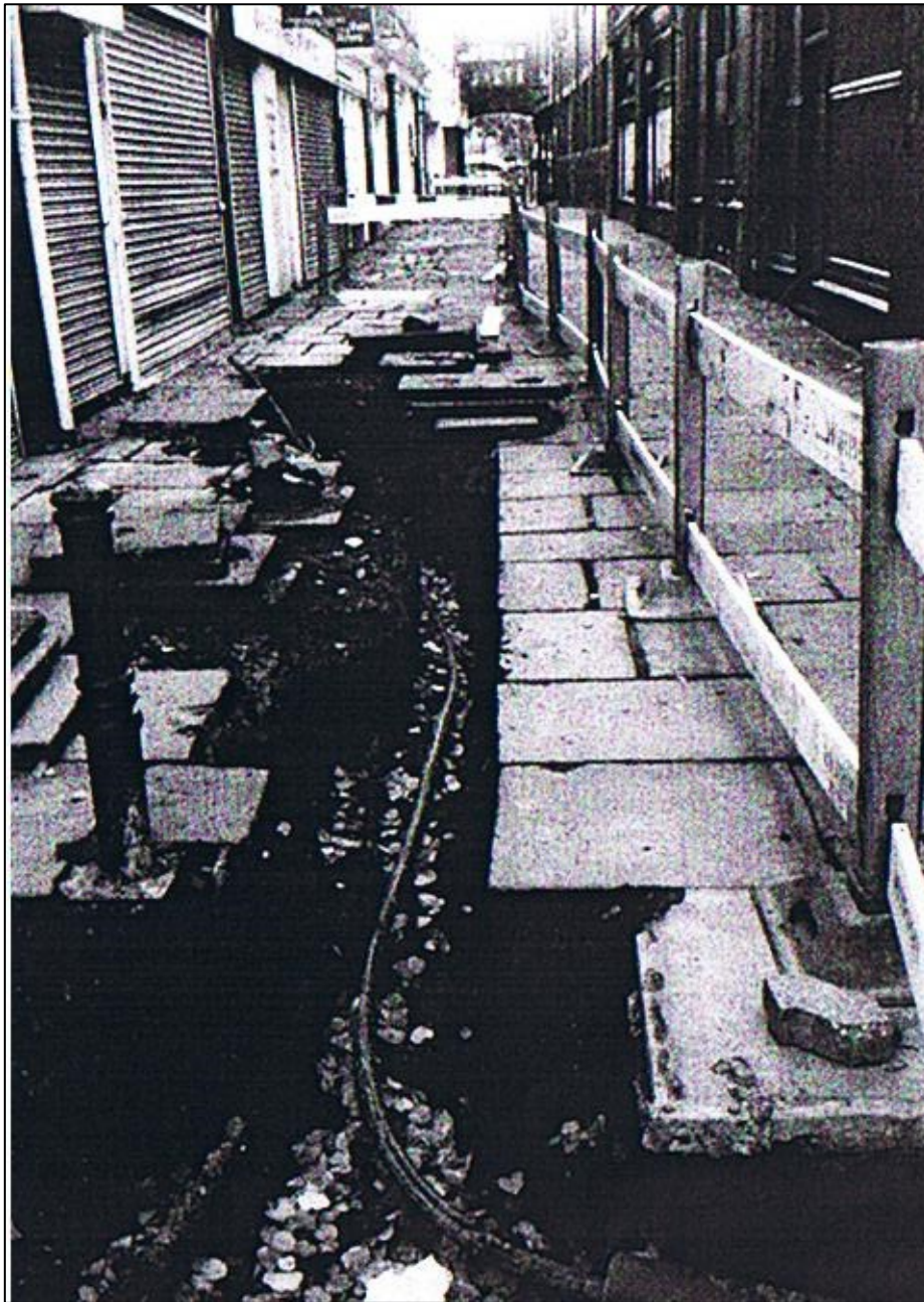
Figure 5. Watching brief when cable laid in 2010
