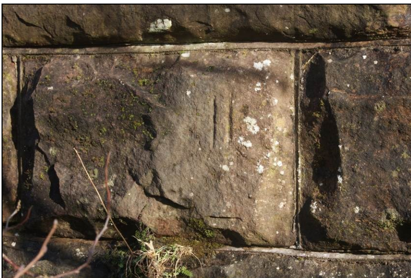
Figure 23. Masonry mark, Pier 2
