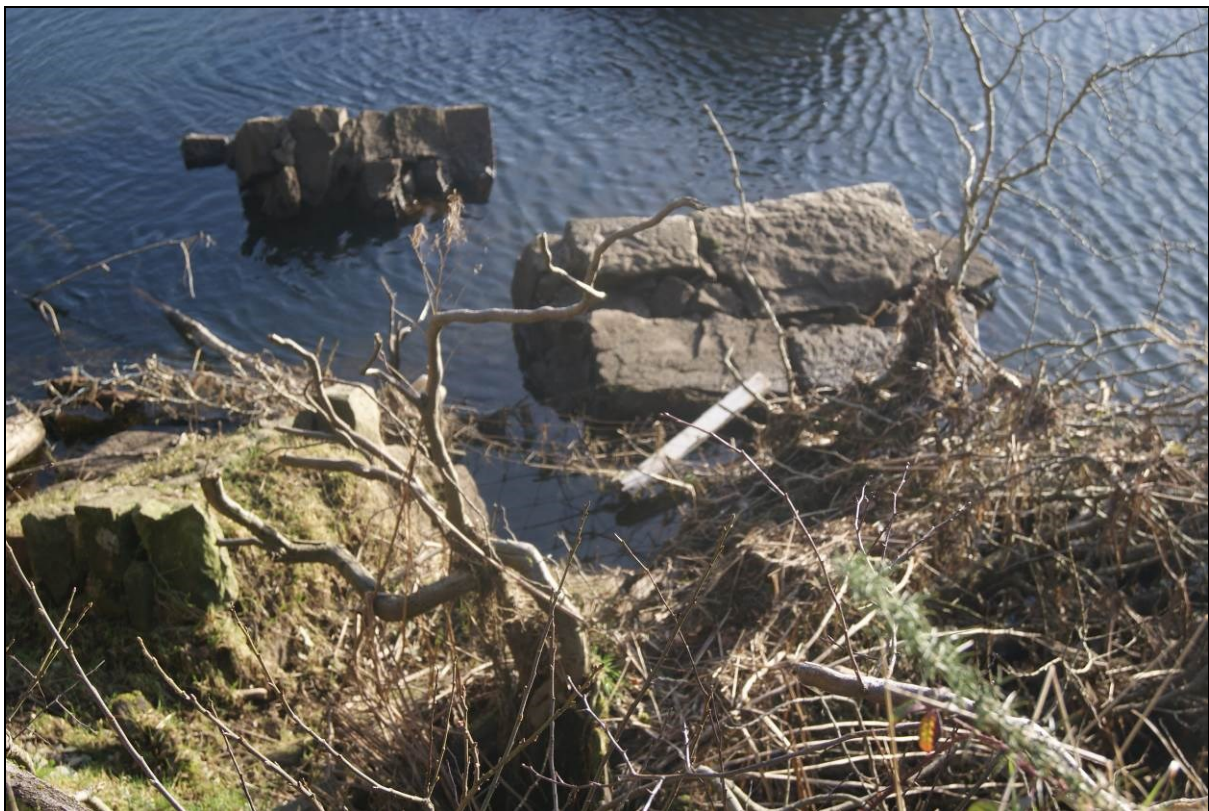
Figure 13. Remnant masonry blocks that had formed the western bridge abutment
