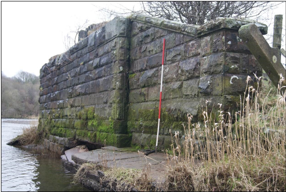
Figure 39. Western elevation forming the eastern bridge abutment.
