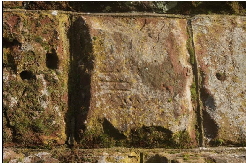
Figure 28. Masonry marks on western elevation on Pier 3
