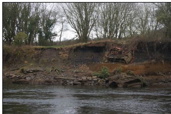
Figure 48. Location of former western abutment
