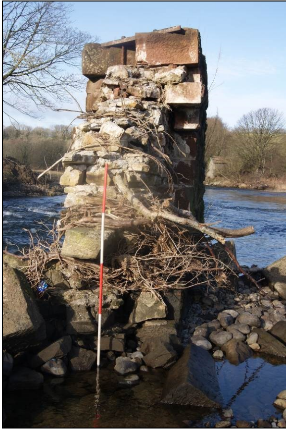
Figure 32. Southern elevation, Pier 5
