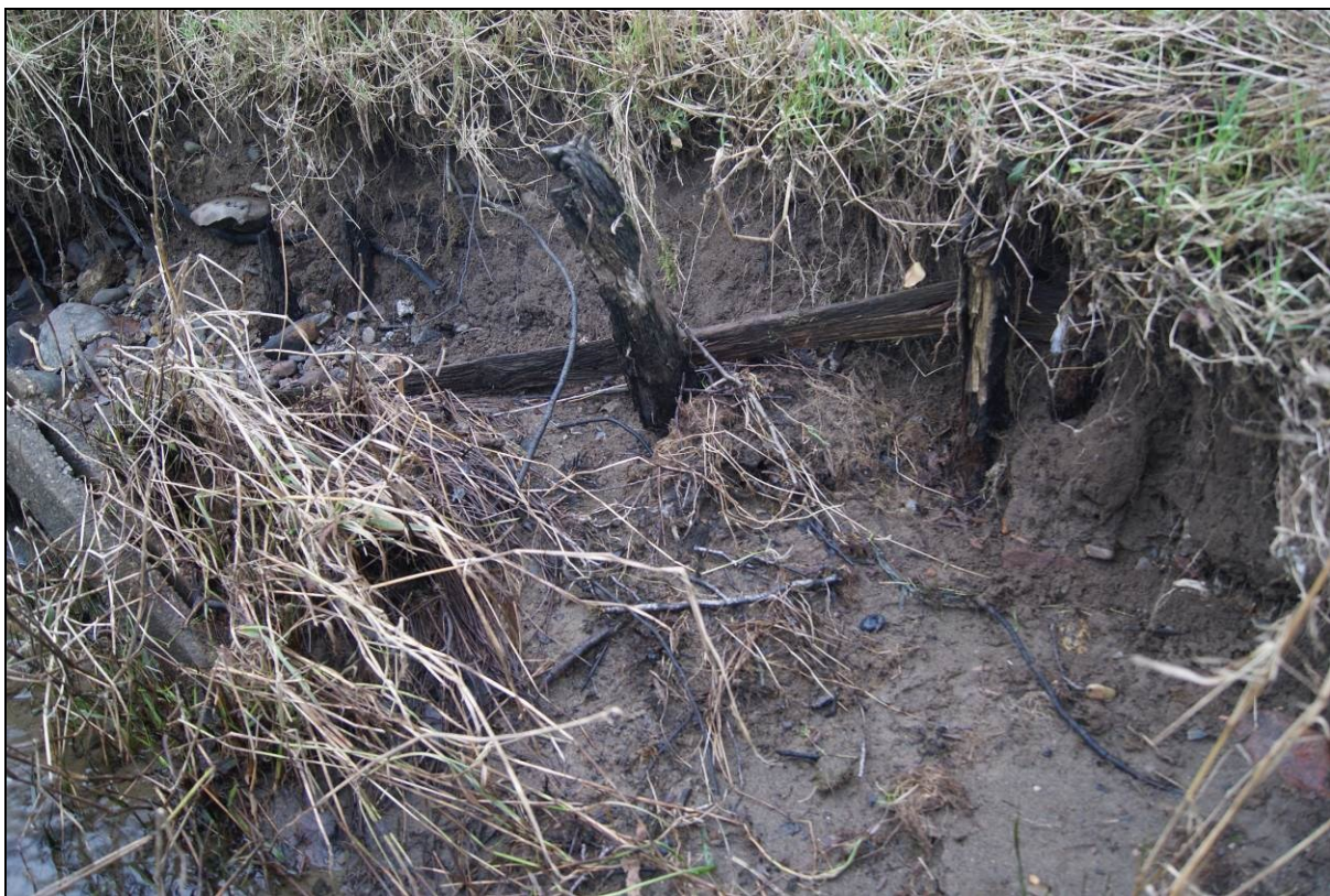
Figure 43. Timber posts and cross member indicating probable earlier timber bridge abutment
