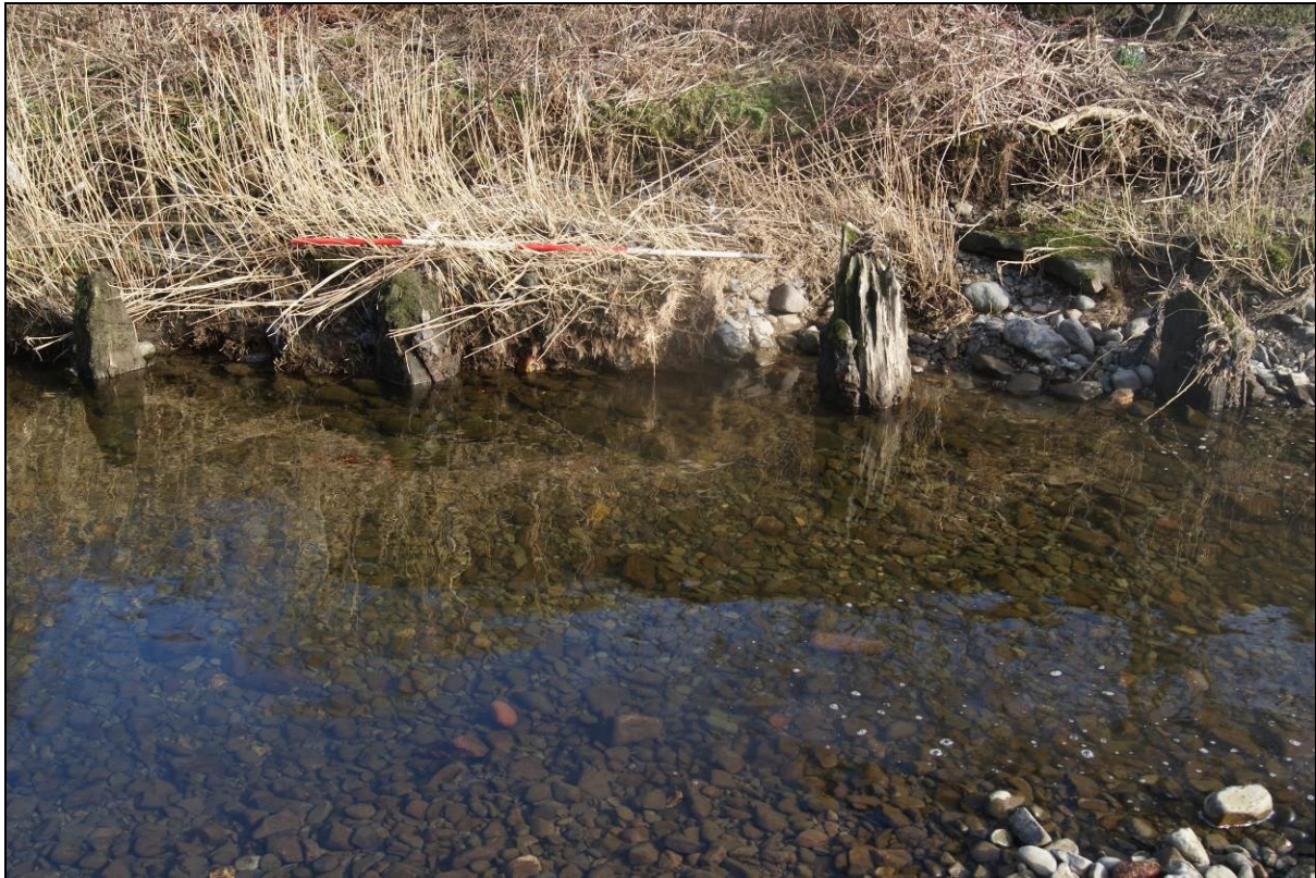
Figure 25. Alignment of four timber piles representing the earlier bridge
