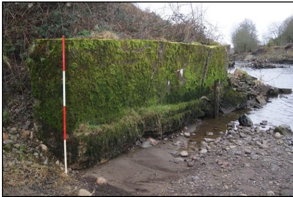
Figure 41. Extant concrete wall built in 1922
