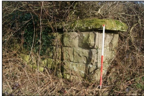
Figure 20. Pier at southern end of east abutment
