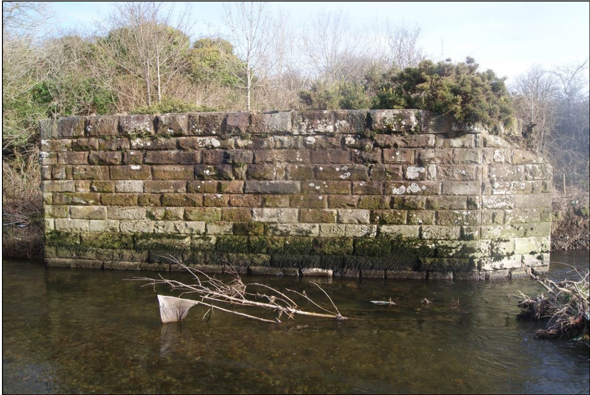
Figure 21. Western elevation illustrating Pier 1
