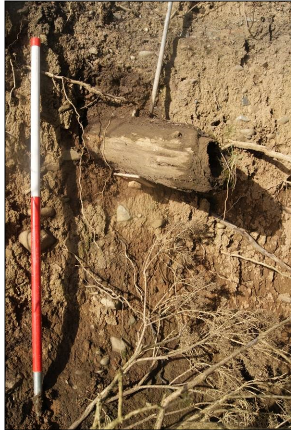
Figure 16. Stanchion base for telegraph pole
