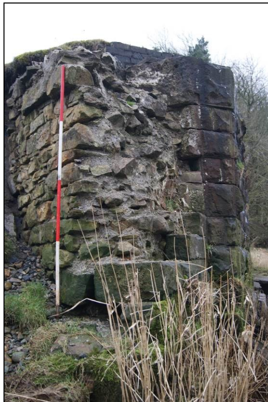
Figure 40. Cross-section through bridge abutment fabric
