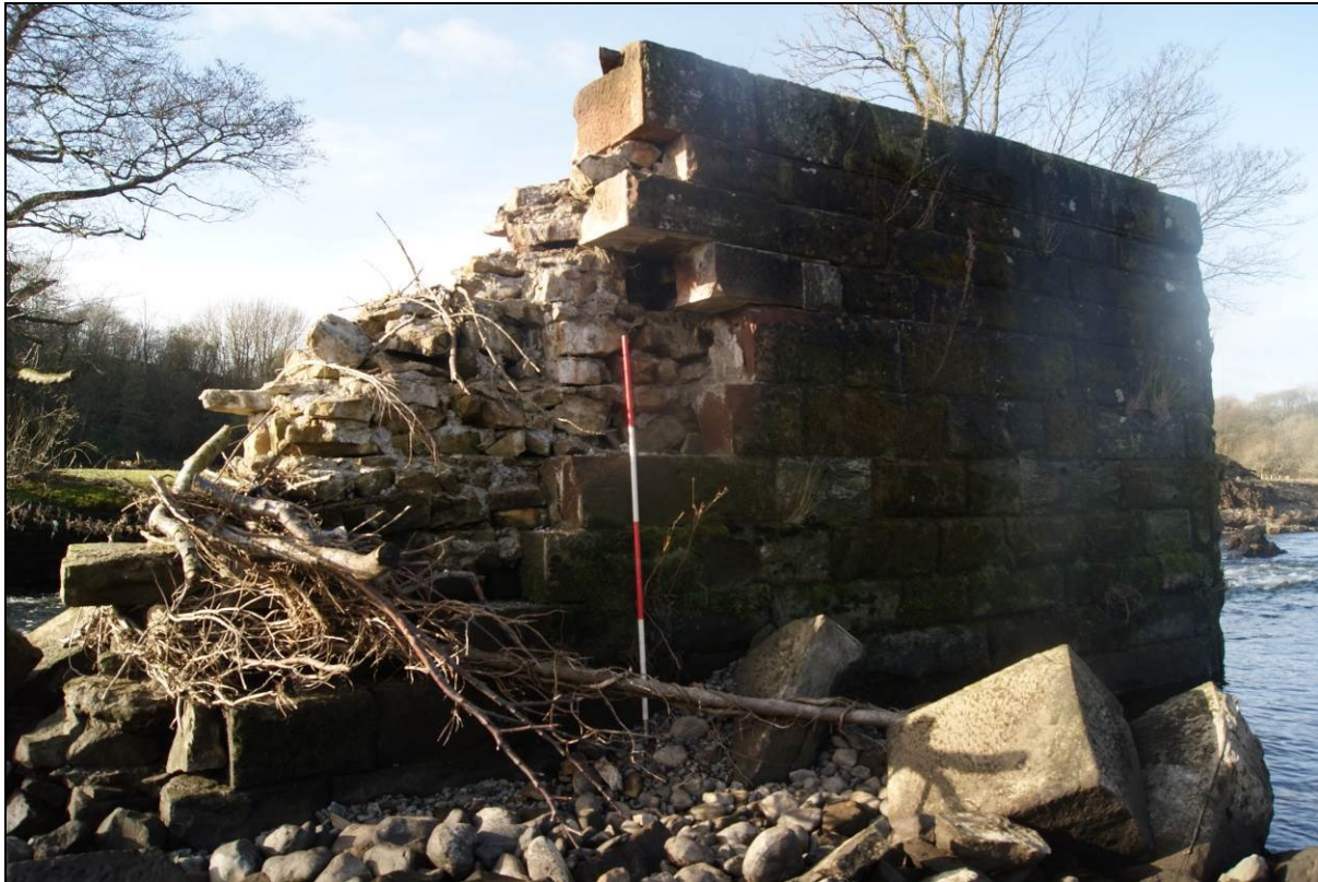
Figure 31. Pier 5 showing eastern elevation
