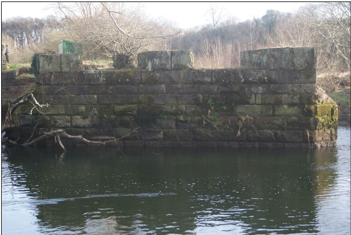
Figure 12. Pier 1, north-western facing elevation
