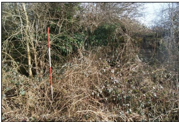
Figure 19. Eastern abutment Ribton Bridge
