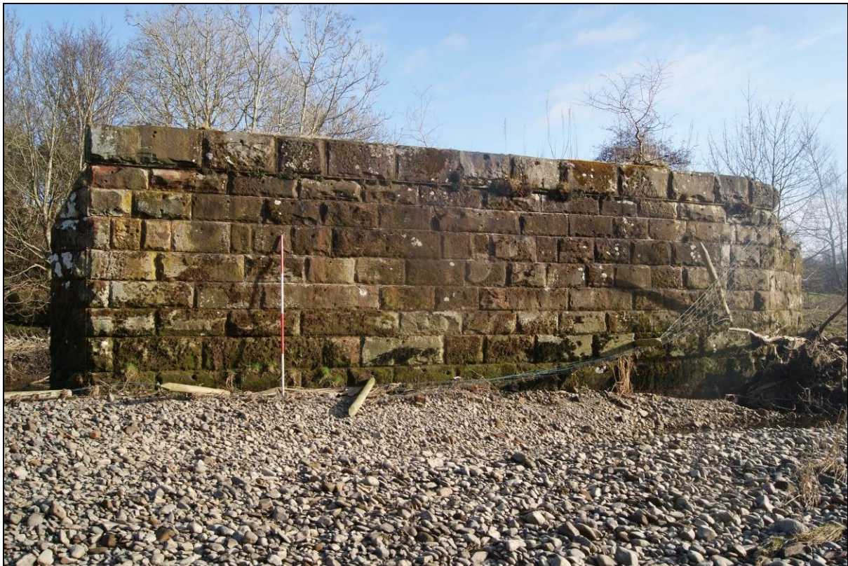
Figure 26. Western elevation of Pier 3
