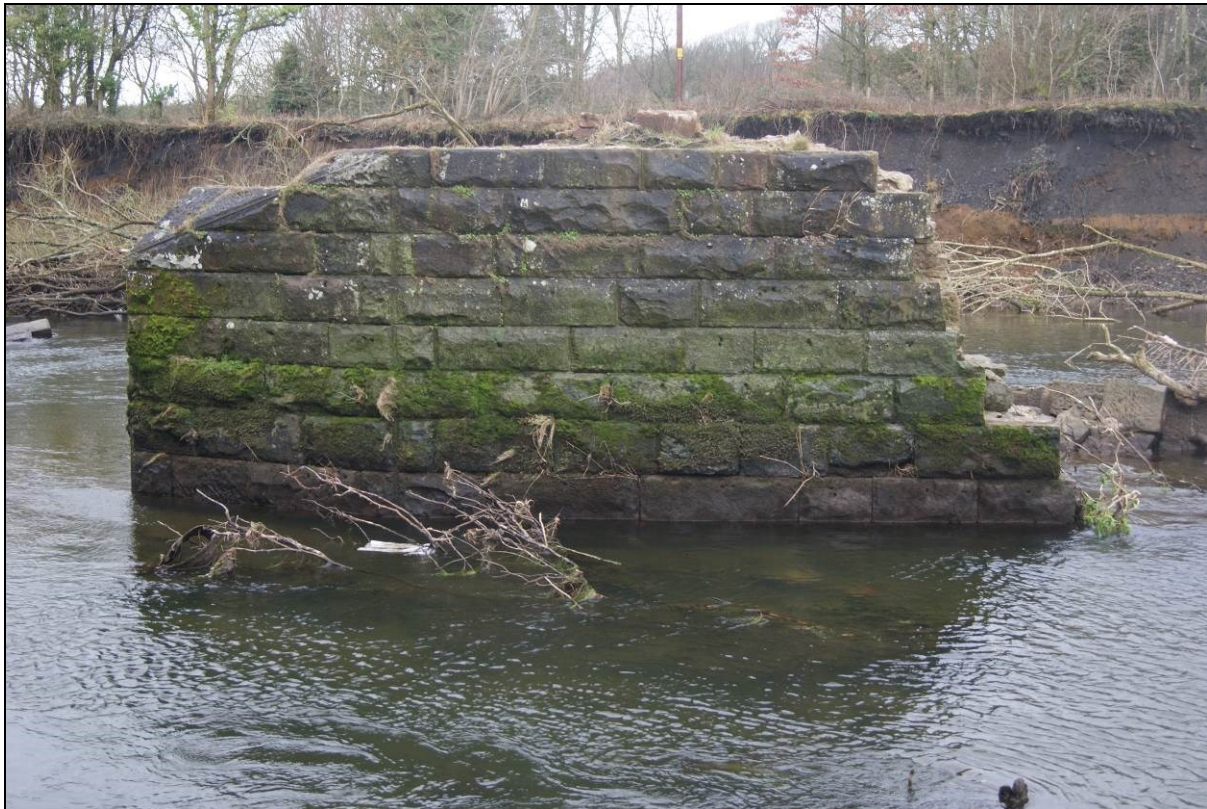
Figure 46. Southern elevation of Pier 1, Camerton Bridge
