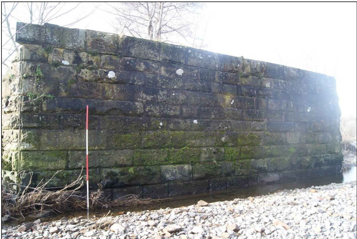
Figure 22. Pier 2 showing the eastern elevation
