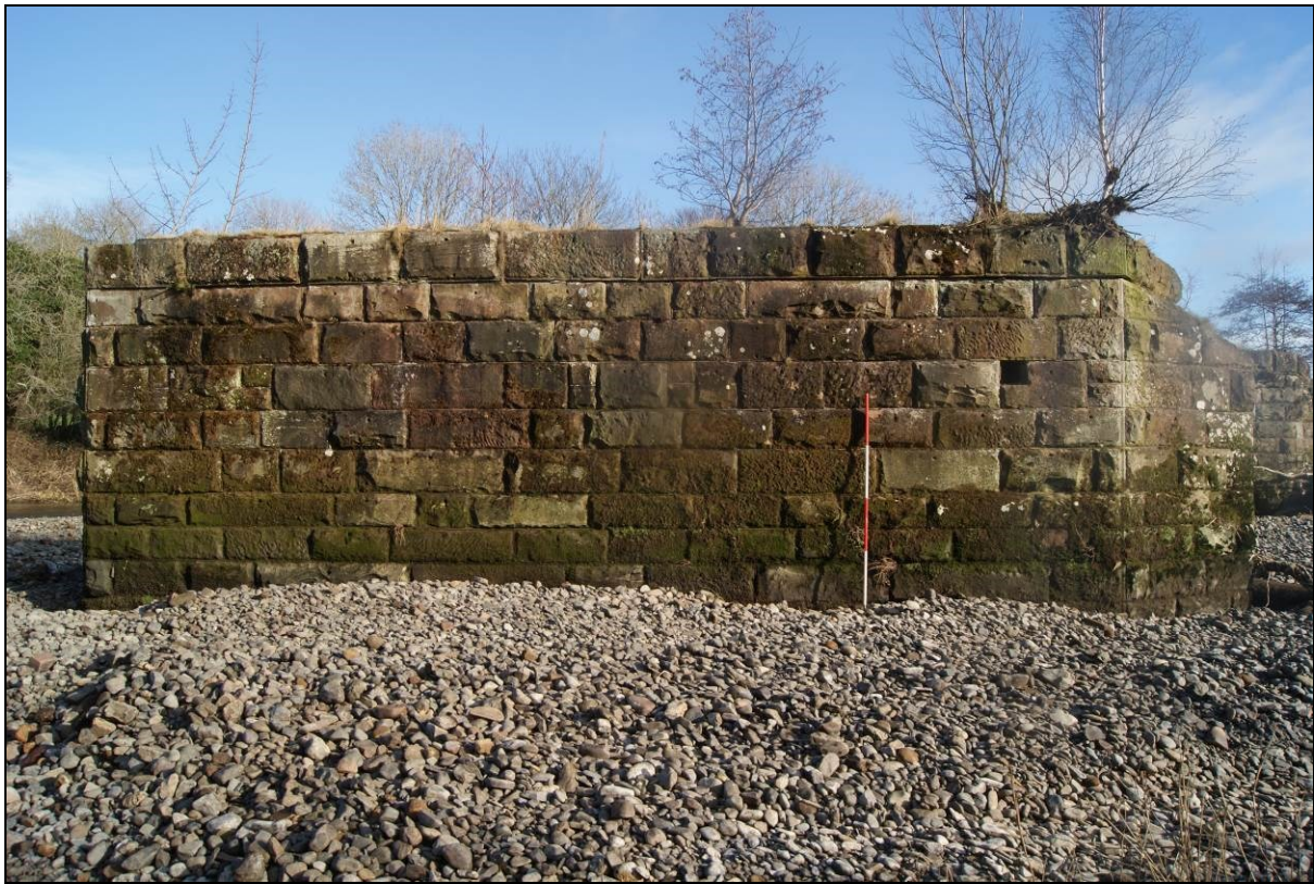
Figure 29. Western elevation of Pier 4, the masonry marks are dead centre
