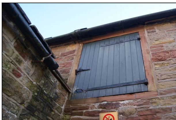
Figure 25. Building 3 butting Building 1
