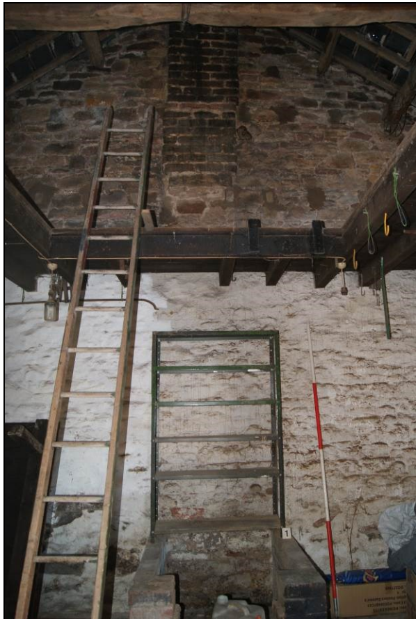
Figure 15. Chimney stack in Building 1
