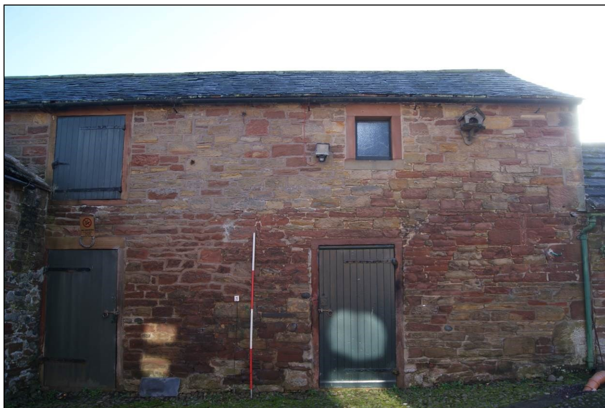
Figure 7. Northern elevation Building 1
