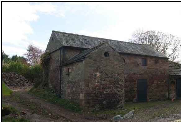
Figure 23. North elevation, Building 3
