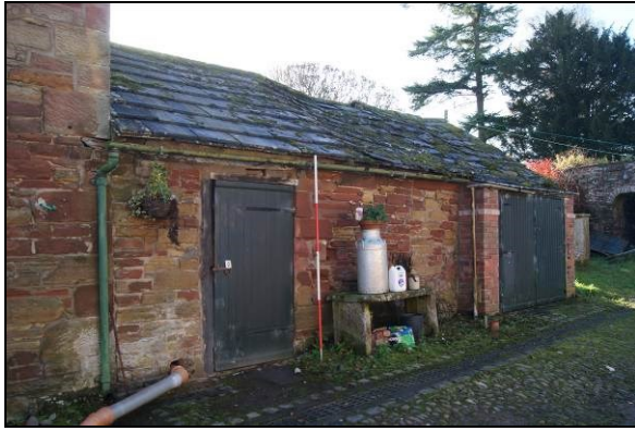
Figure 19. Northern elevation Building 2
