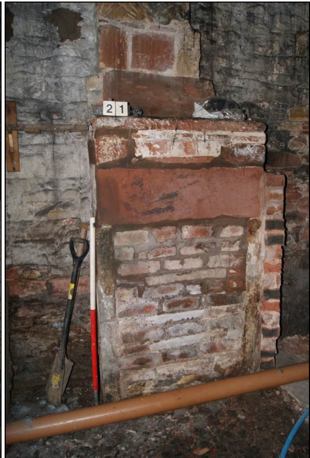
Figure 16. Fireplace, Room 1, Building 2
