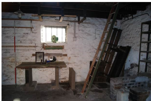
Figure 10. Interior of Room 2, Building 1
