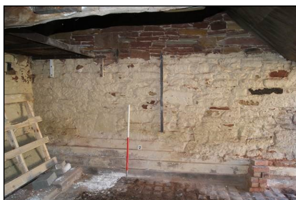
Figure 17. Internal area Room 2, Building 2
