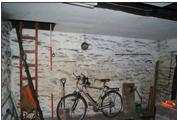
Figure 9. Interior of Room 1, Building 1
