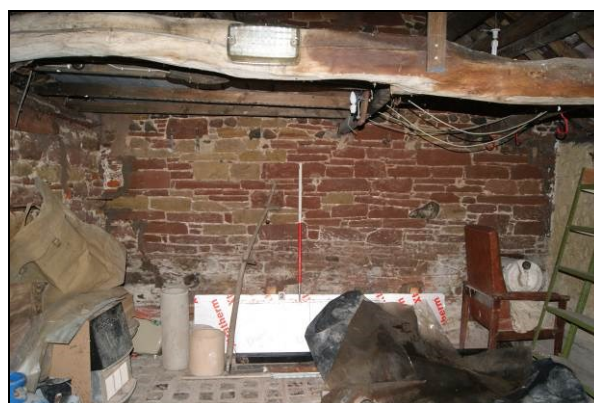
Figure 18. Sandstone partition wall Building 2
