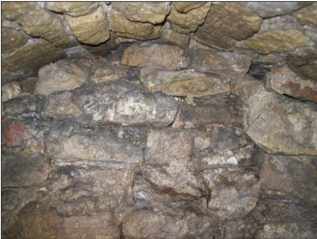
Figure 12 - Blocked Rear Wall in Cellar (Southern Vault)
