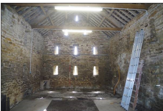
Figure 10. Gable end of threshing barn
