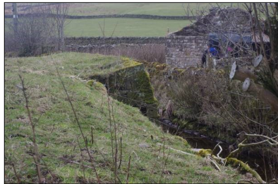
Figure 16. Bridge abutment for possible Wall
