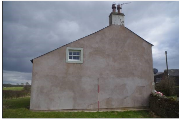
Figure 7. Outshut housing staircase
