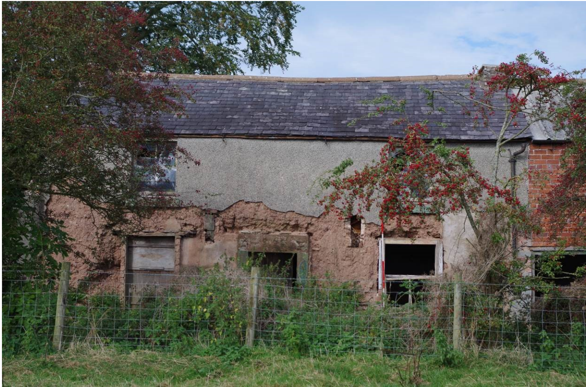
Figure 52. Clay dabbins cottage, southern elevation
