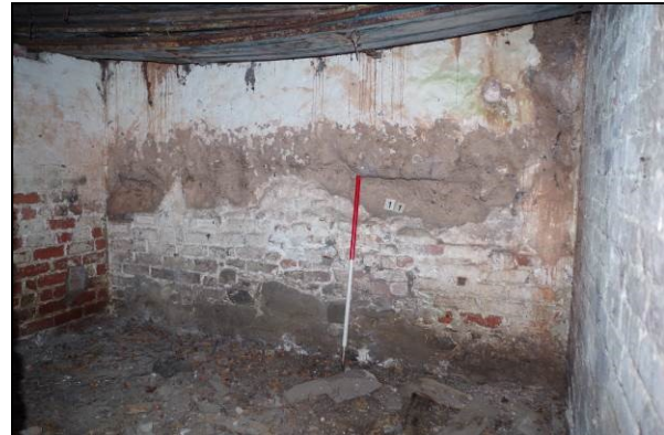
Figure 34. Interior of stall 5, Room 11
