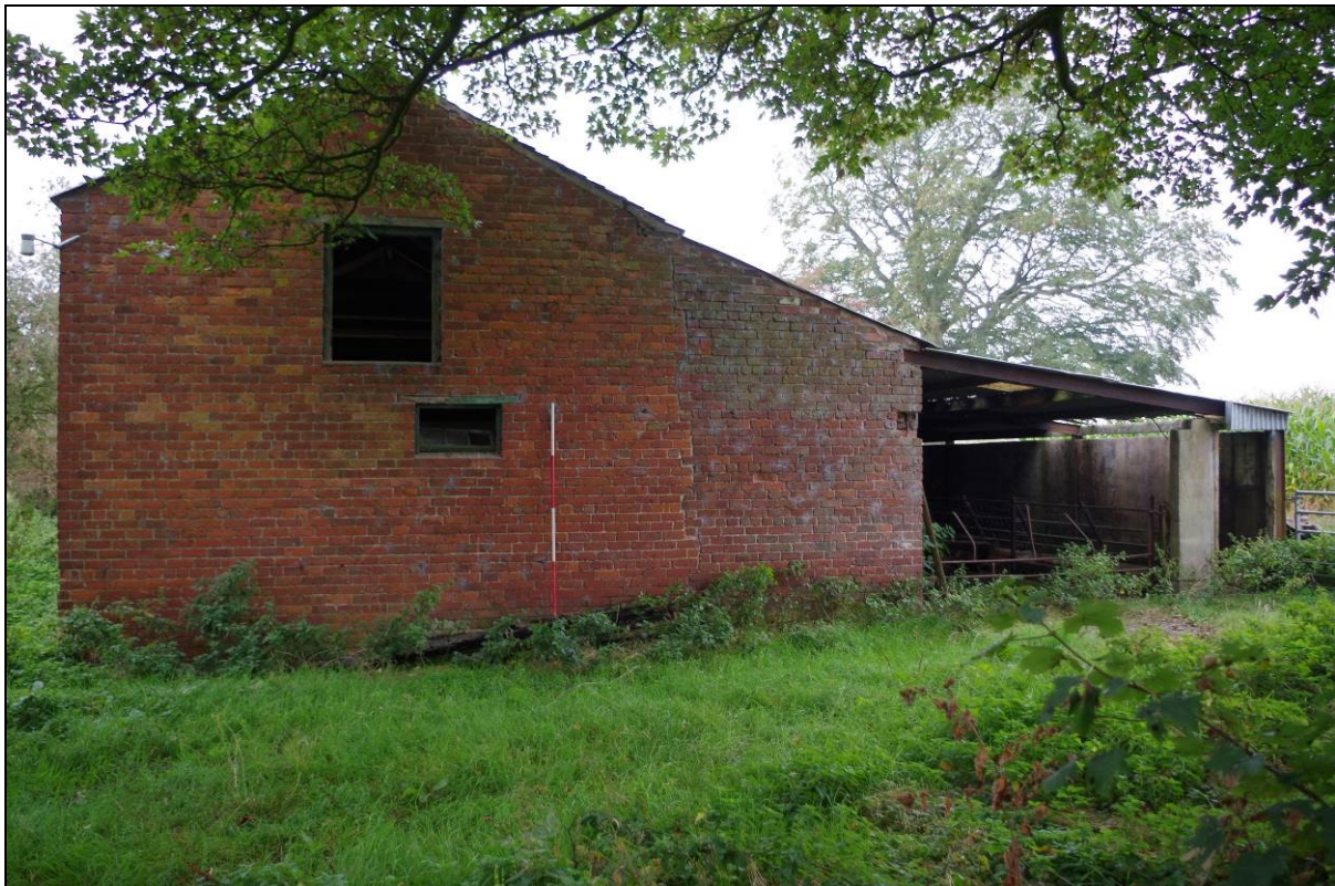
Figure 57. Barn and shed, eastern elevation
