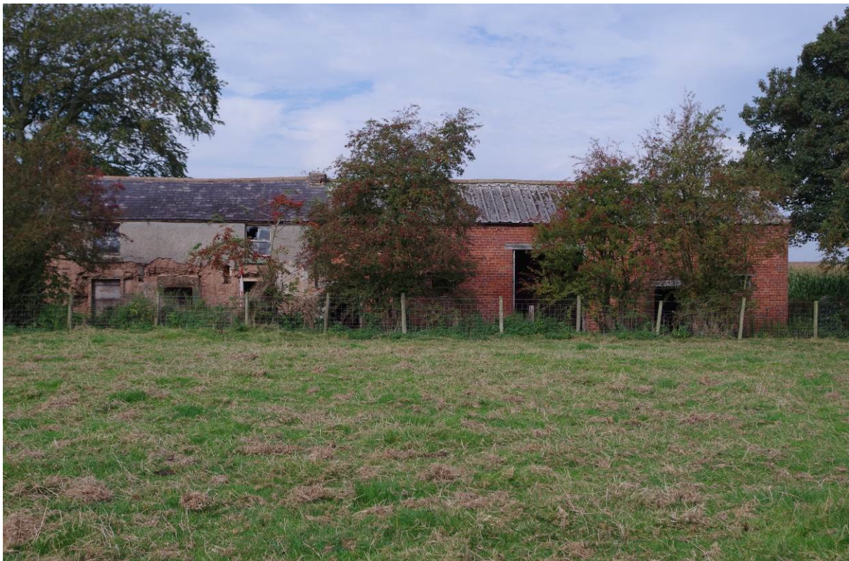
Figure 53. Brick barn southern elevation
