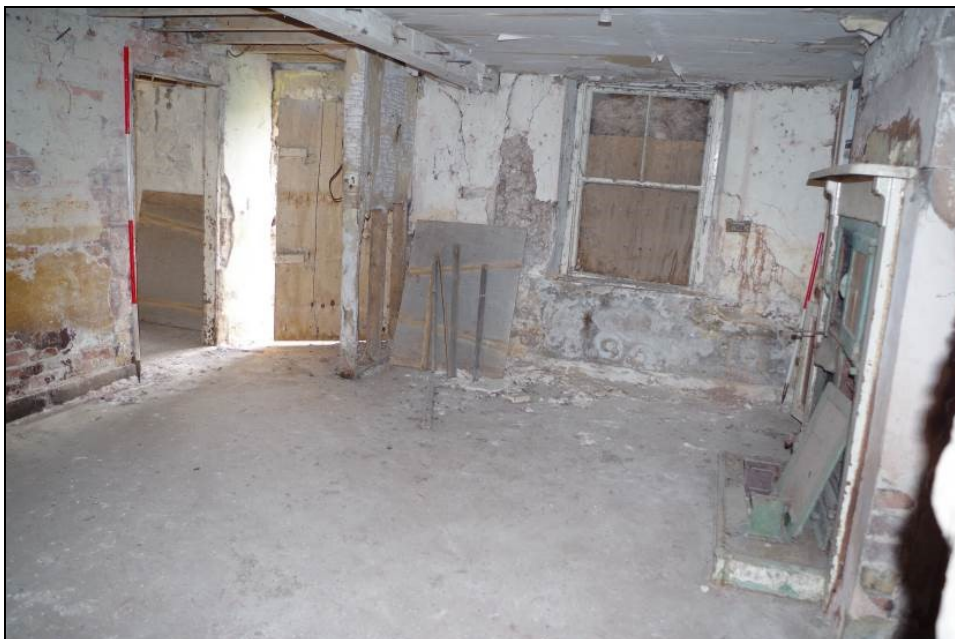
Figure 8. Interior of Room 1
