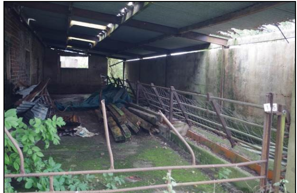
Figure 38. Interior of lean-to, Room 15
