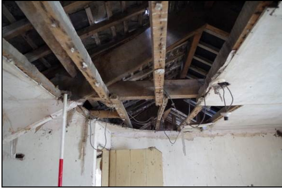
Figure 43. Exposed roof and cruck blade
