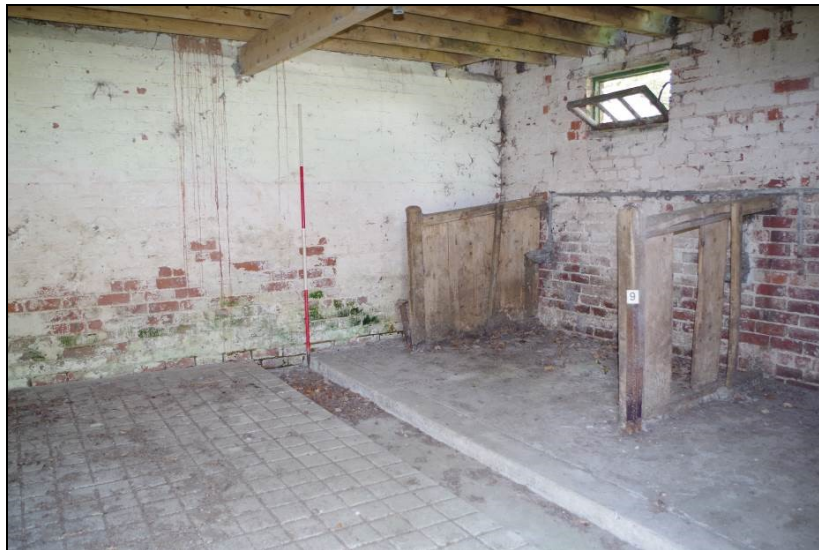
Figure 32. Interior of stall 3, Room 9
