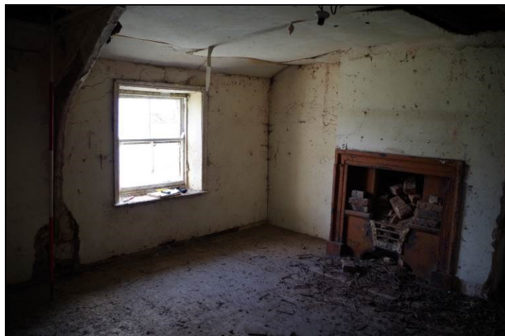
Figure 42. Interior of Room 5
