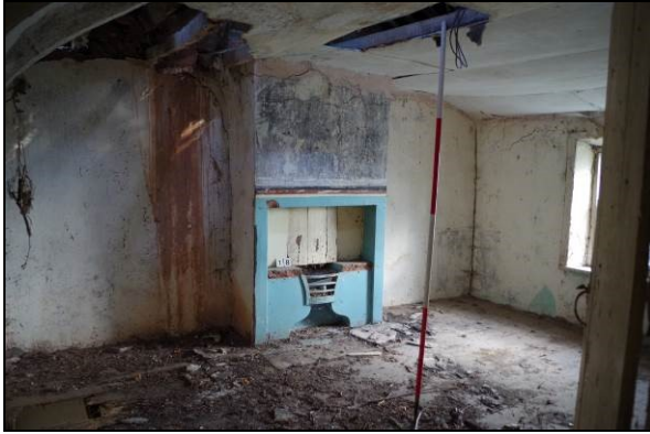
Figure 47. Interior of Room 18
