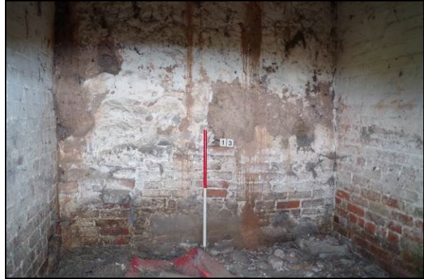
Figure 36. Interior of stall 7, Room 13
