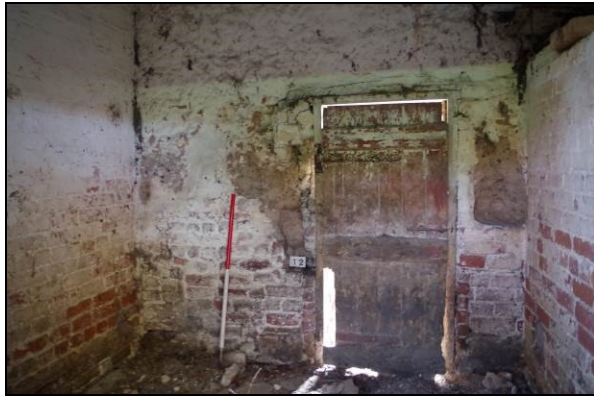
Figure 35. Interior of stall 6, Room 12
