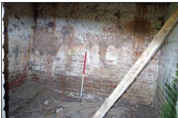
Figure 37. Interior of stall 8, Room 14
