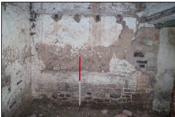
Figure 33. Interior of stall 4, Room 10
