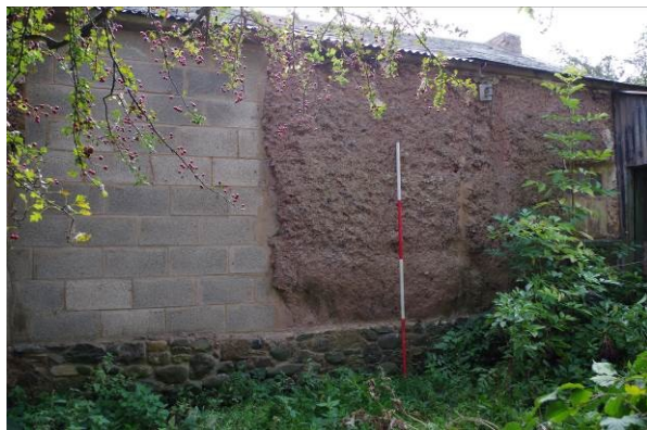
Figure 27. Exterior wall showing modern repair
