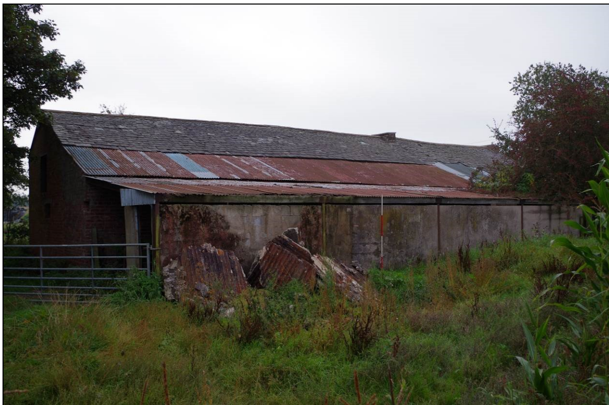
Figure 55. Barn and shed, northern elevation
