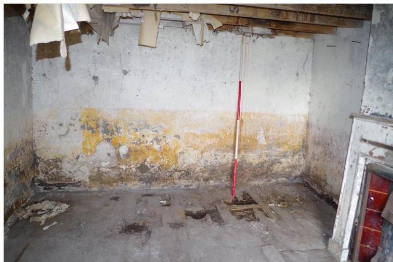
Figure 15. Interior of Room 2
