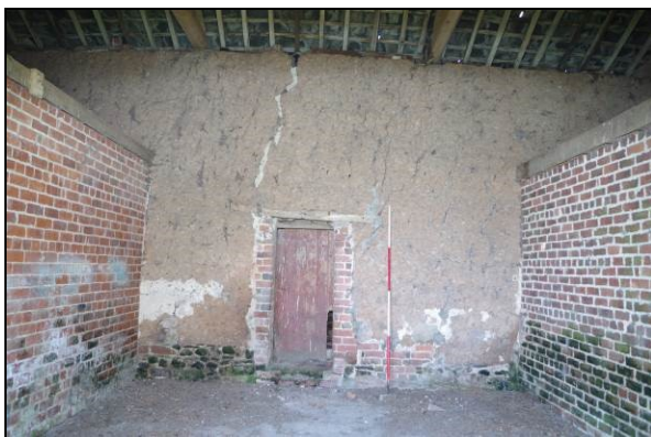
Figure 30. Interior of threshing barn
