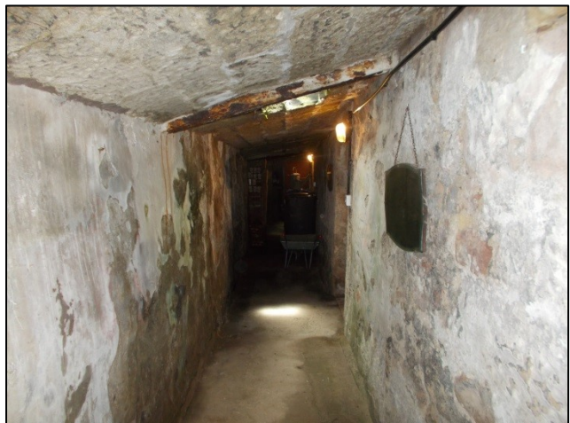
Figure 5. Passage between defences and 23 Quay Walls
