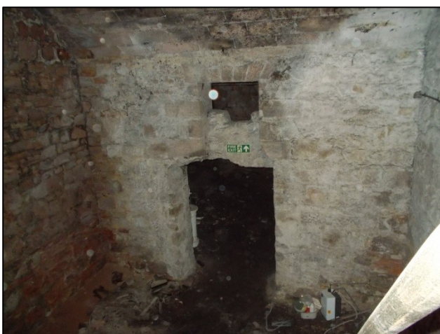
Figure 4. Cellar within 18 Quay Walls
