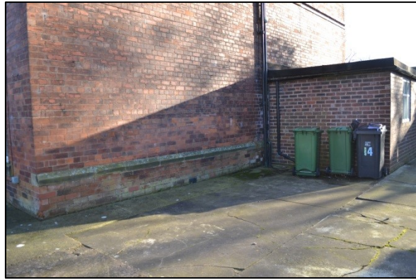
Figure 8. Former outbuilding and concrete drive
