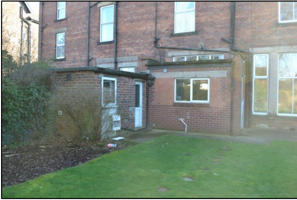
Figure 7. Former kitchen in Area 1
