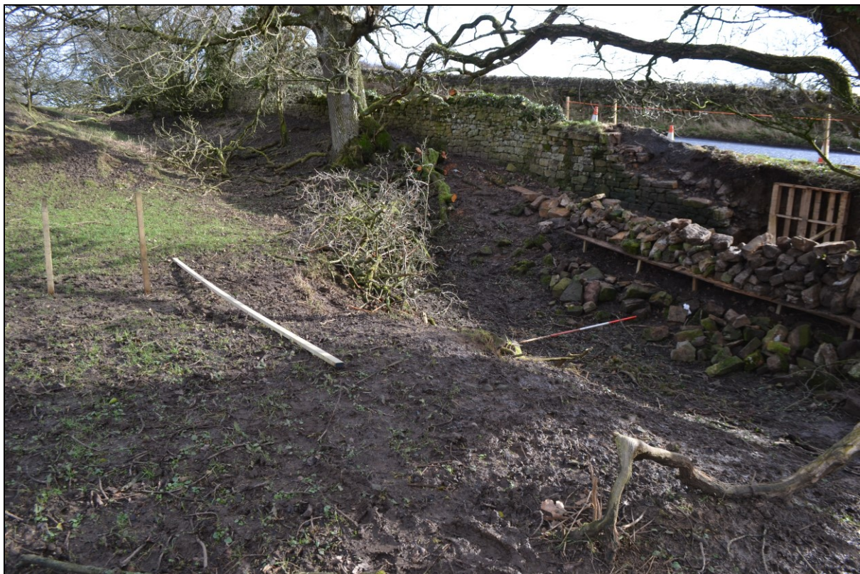
Figure 20. Wall Ditch as at present with the retaining wall
