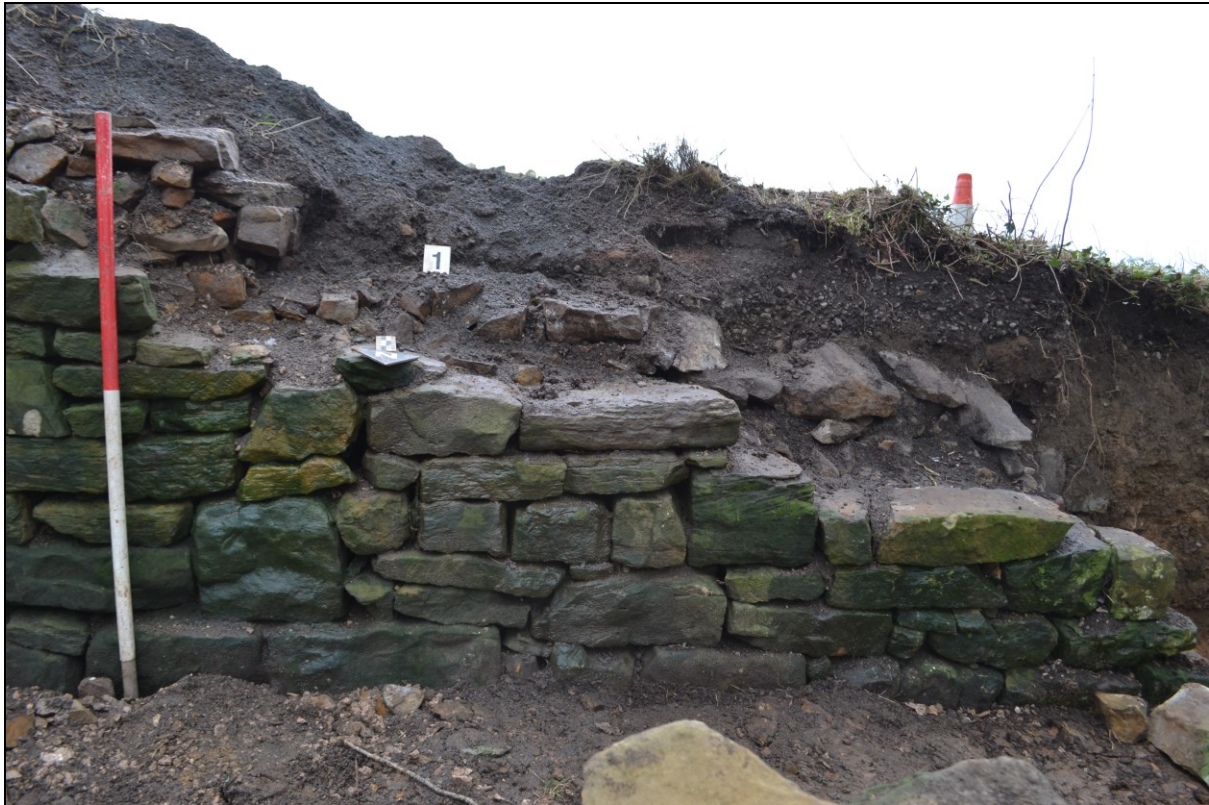
Figure 5. Intervention 1 following removal of loose and extraneous masonry
