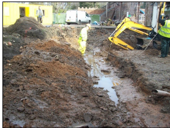
Figure 8. Excavation of footings
