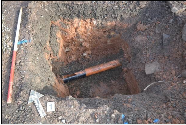
Figure 7. Trench 1 with drain
