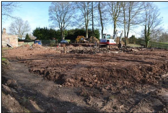
Figure 5. Raised ground level to the south
